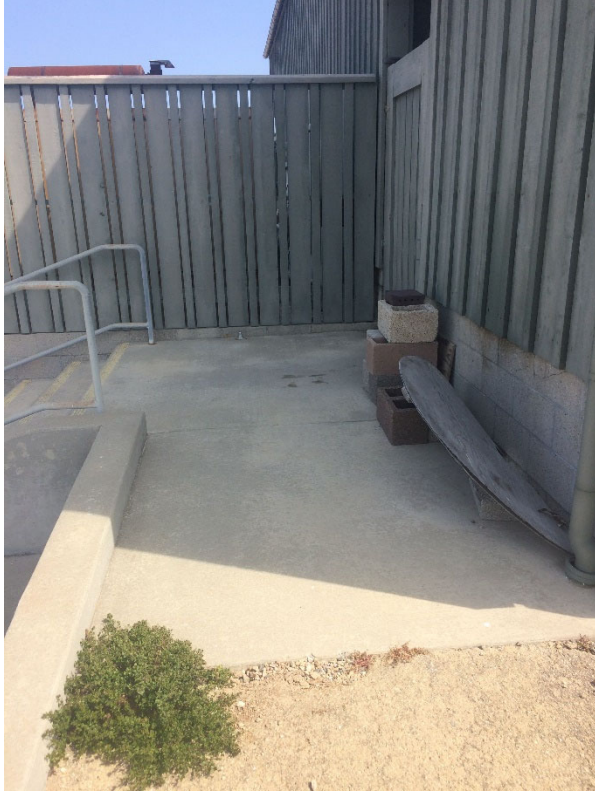
Existing wood fencing at storage yard.
