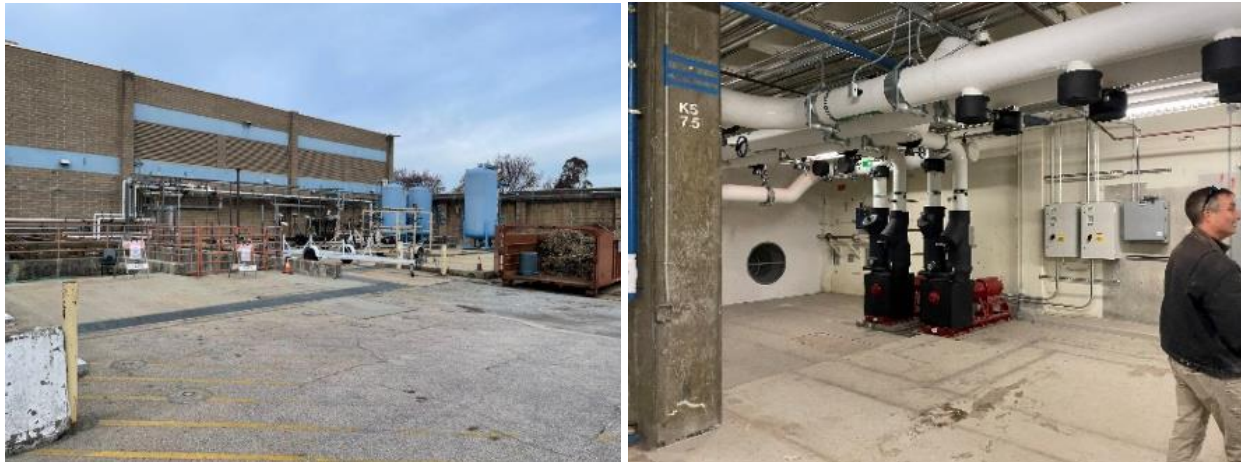
Figure 30 – Loading dock/ pump room
