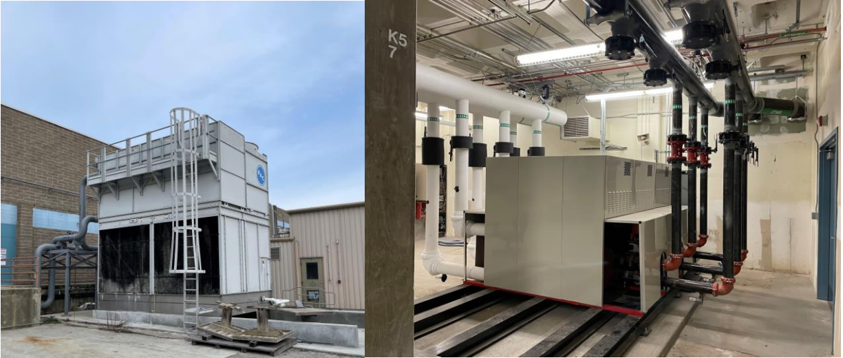
Figure 31 – Existing cooling tower and chillers
