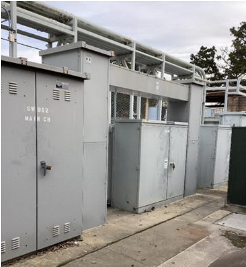
Figure 41 – Westside Research Park
