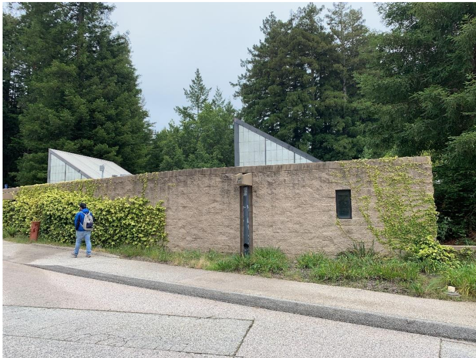
Slope on west elevation (Looking east from the street)
