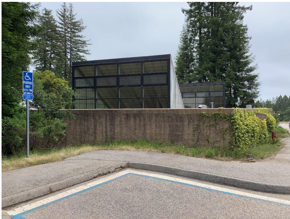
Northwest corner (Looking southeast)
