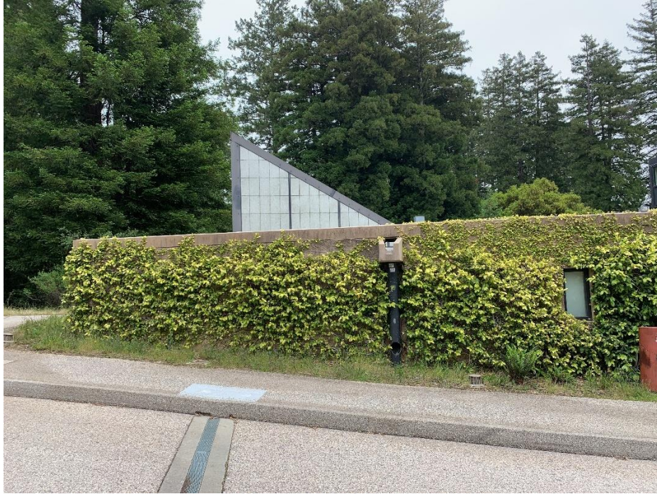
Partial west elevation (looking east)
