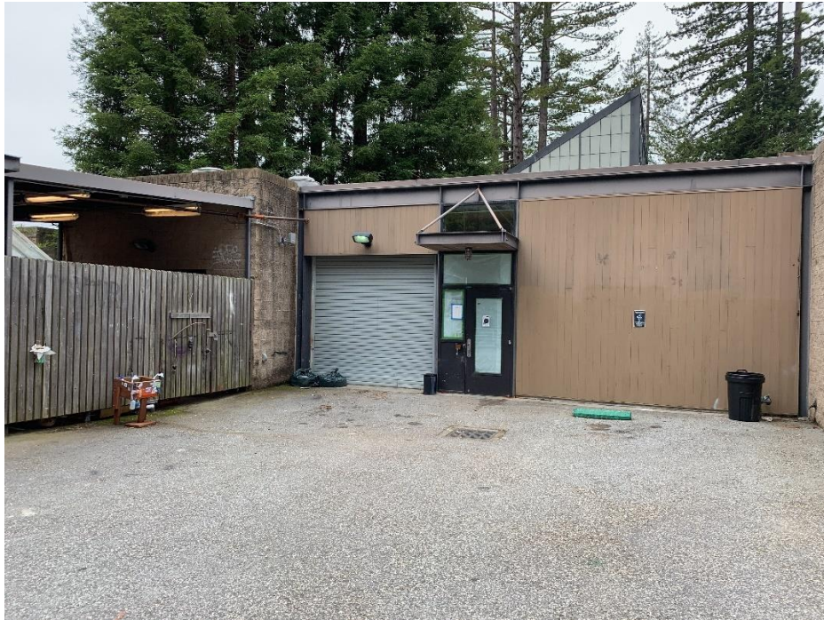
Partial east elevation (looking west at the ceramic workshop)
