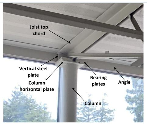
Close-up of the joist-to-column connection
