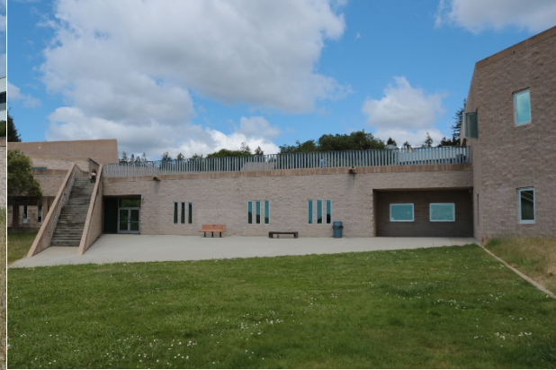
South View of Practice Studios and Class Lab
