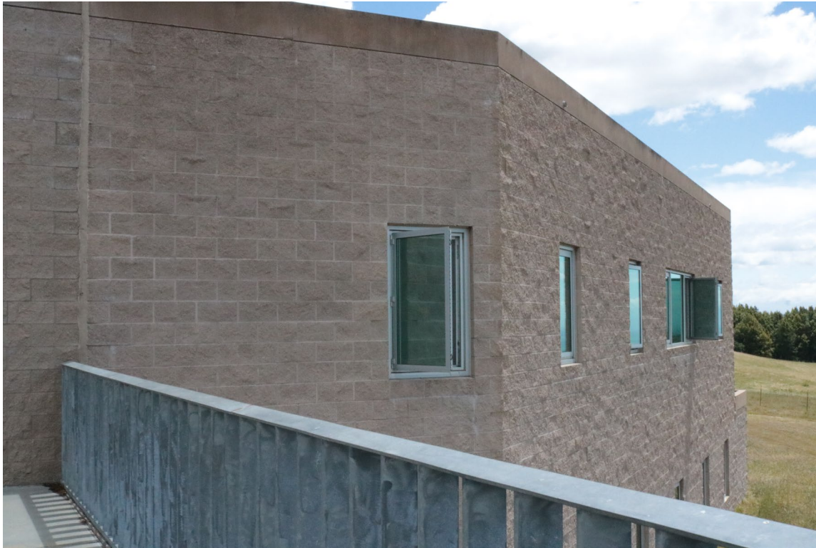
Expansion joint at Building 3W, looking south
