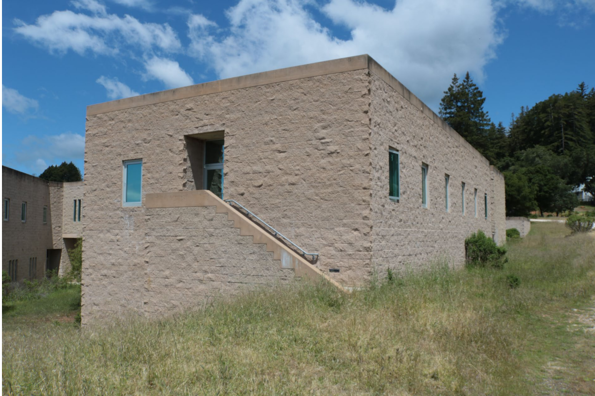
South elevation of Building 3E looking north
