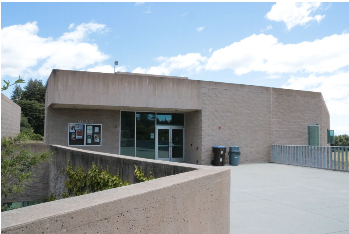
Transition from CAAN 7922 to Building 3W at Level 2 entrance, looking east
