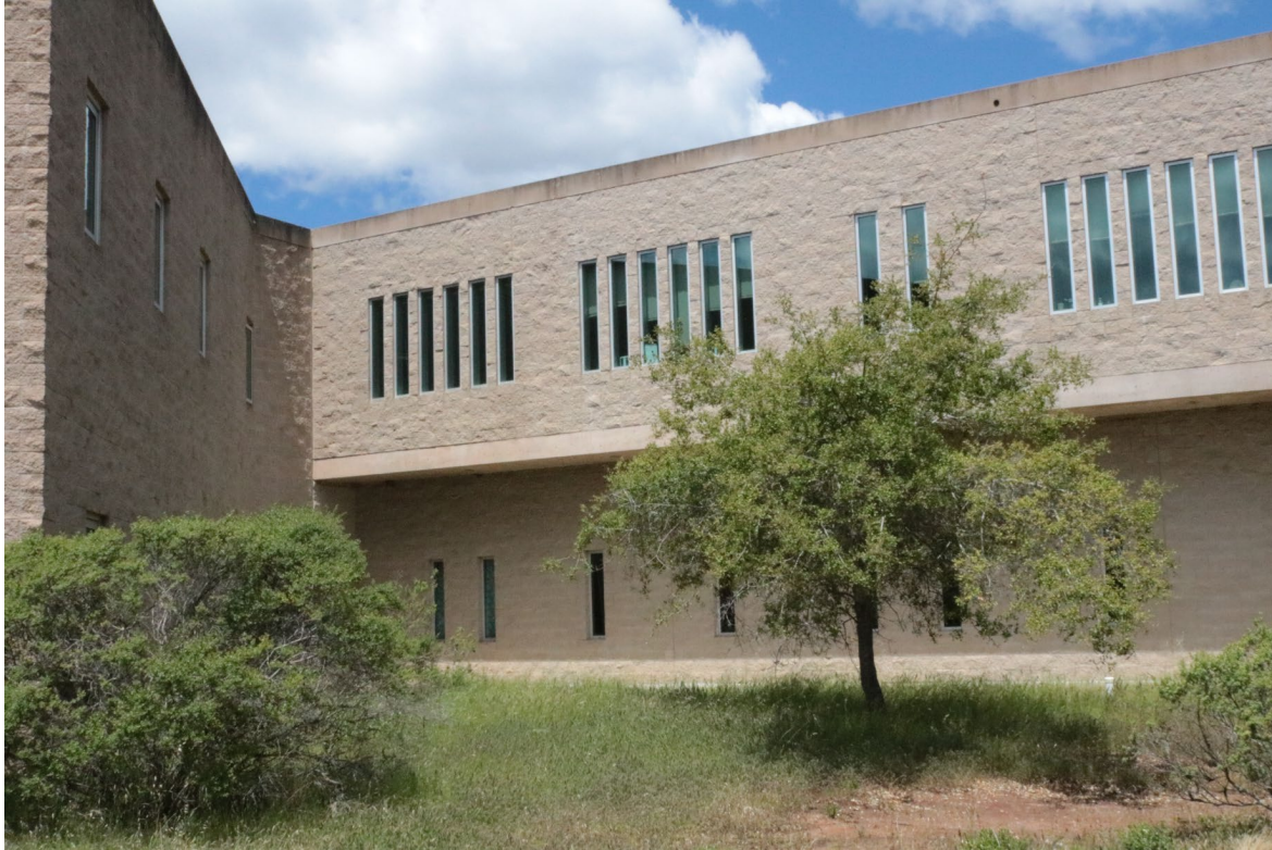
East elevation of Building 3W and south elevation of CAAN 7922, looking north
