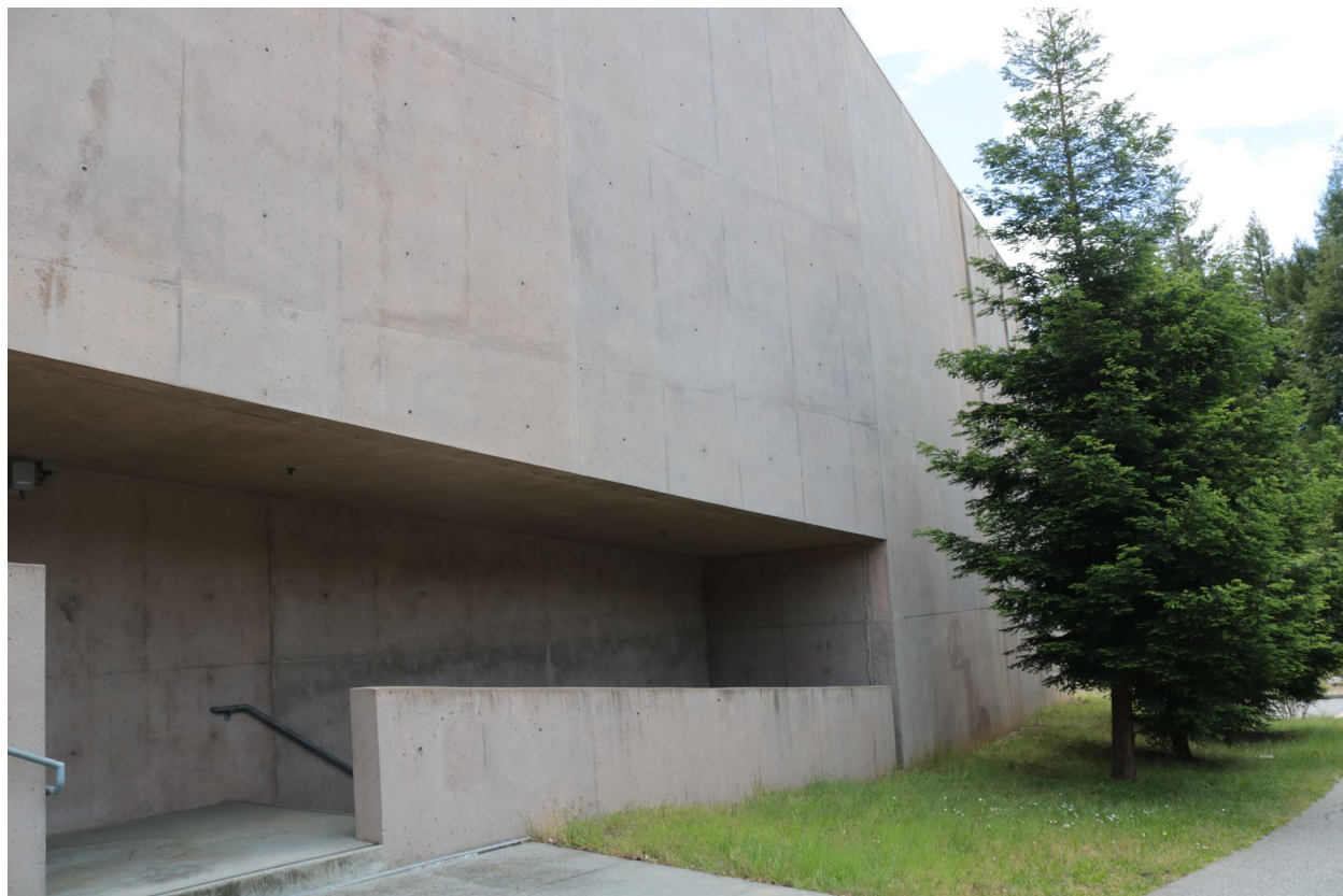
Discontinuous wall at west elevation of Recital Hall (looking north)
