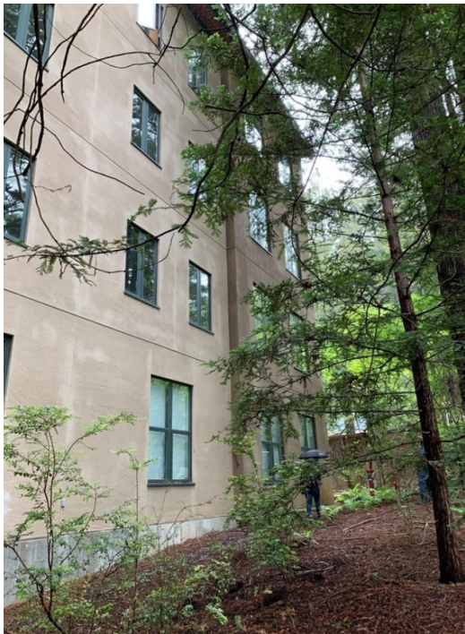
Figure 4 - View of stepped perimeter shear wall (East Elevation)
