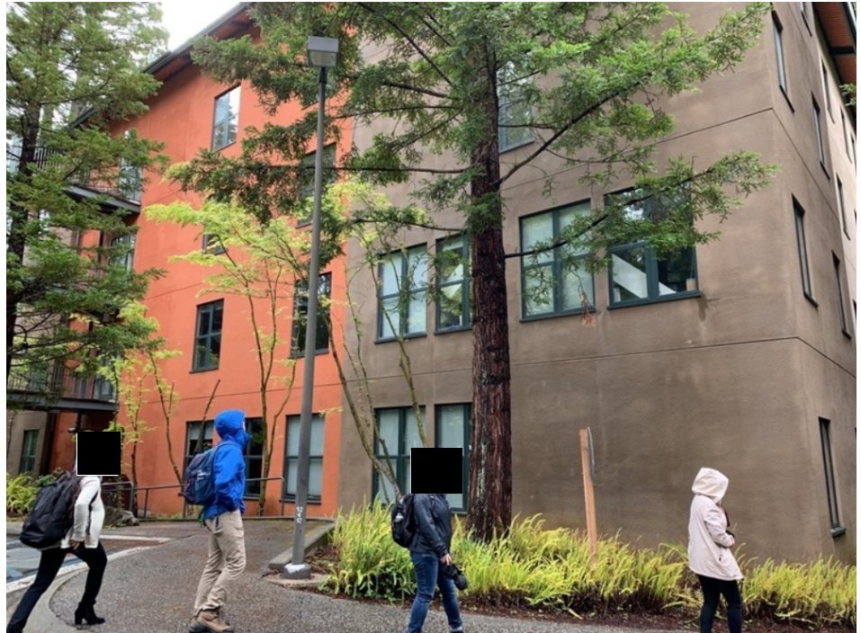
Figure 1 - North Elevation View of the North Tower
