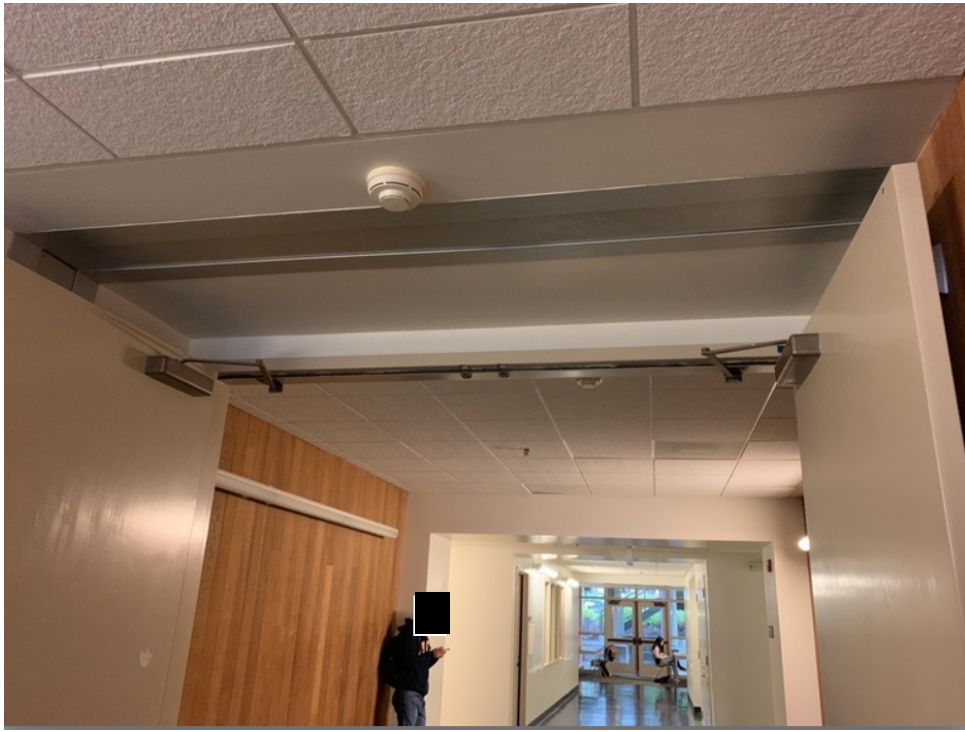
Figure 3 - View of hall way looking toward north. Seismic Joint is seen above the doors.
