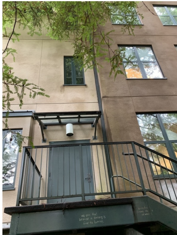
Figure 2 - Seismic Joint between the North and South Towers (North is to the right)
