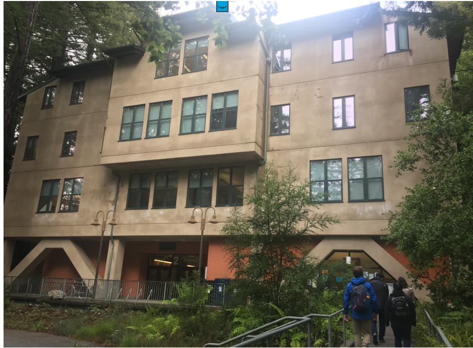
Figure 1 - South Elevation View of the South Tower
