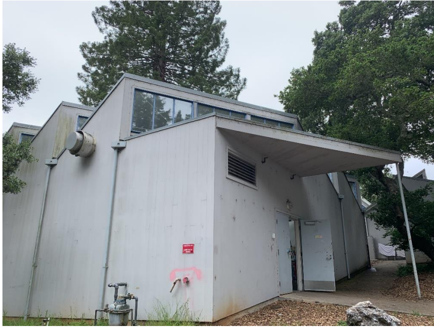
Northeast corner (looking southwest)
