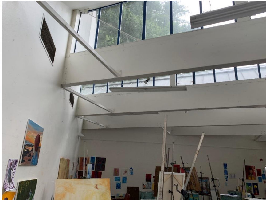
Glulam beams supporting clerestory windows.
