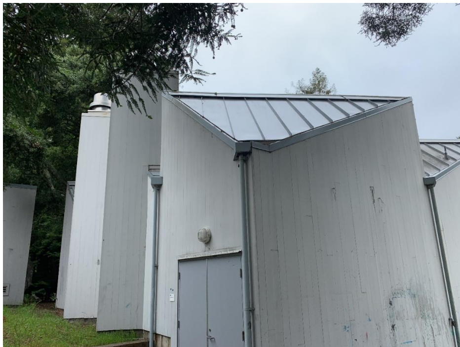
Southwest corner (looking northeast)
