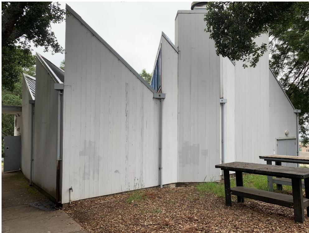
Northwest corner (looking southeast)
