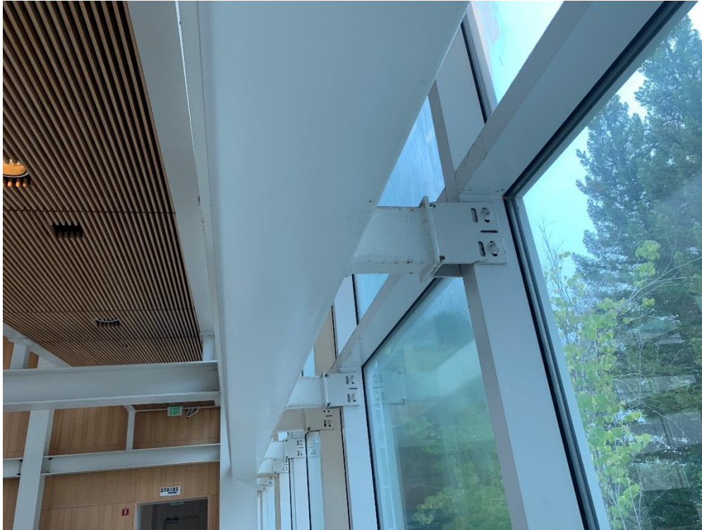
Interior View of Detail at Atrium Window Mullions at North Elevation
