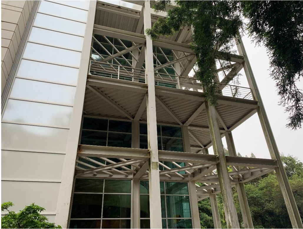
West Elevation Lobby Exposed Framing and Full-Height Glazing at Southwest Corner (Looking Southeast)
