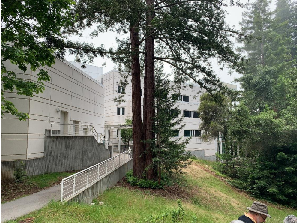
West Elevation Office Block A2 (Center), Lobby (Right), Lecture Hall (Left, Looking Southeast)
