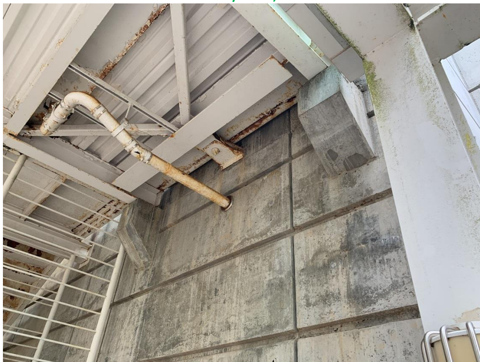
Bridge Anchored to Lab Block D at Right (Looking Northeast)
