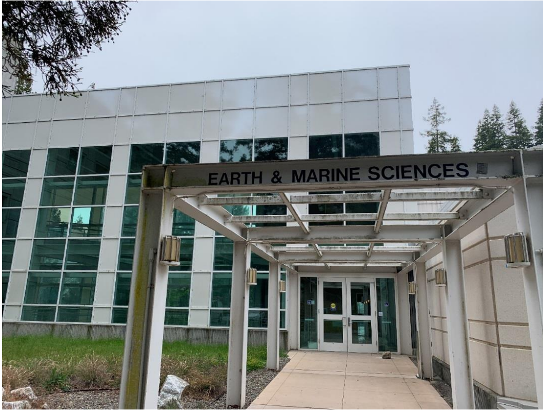
North Elevation with Atrium Entry
