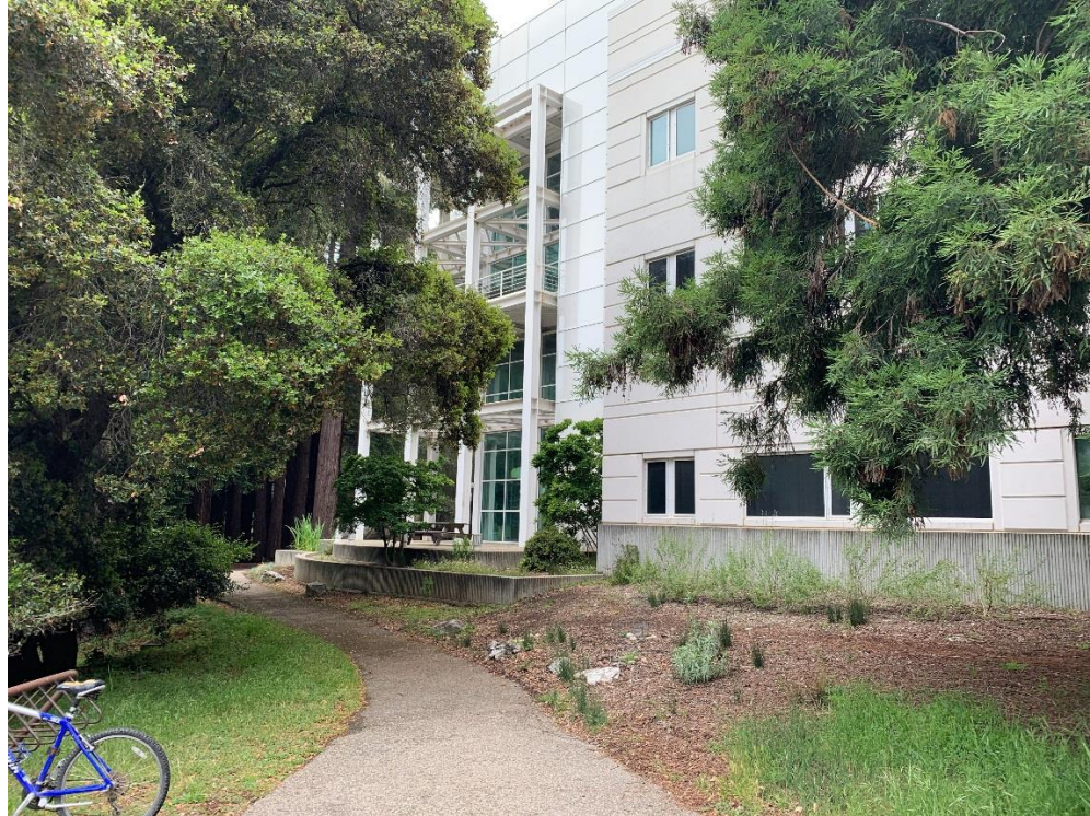
South Elevation Office Block A1 (Right) and Lobby (Left, Looking Northwest)
