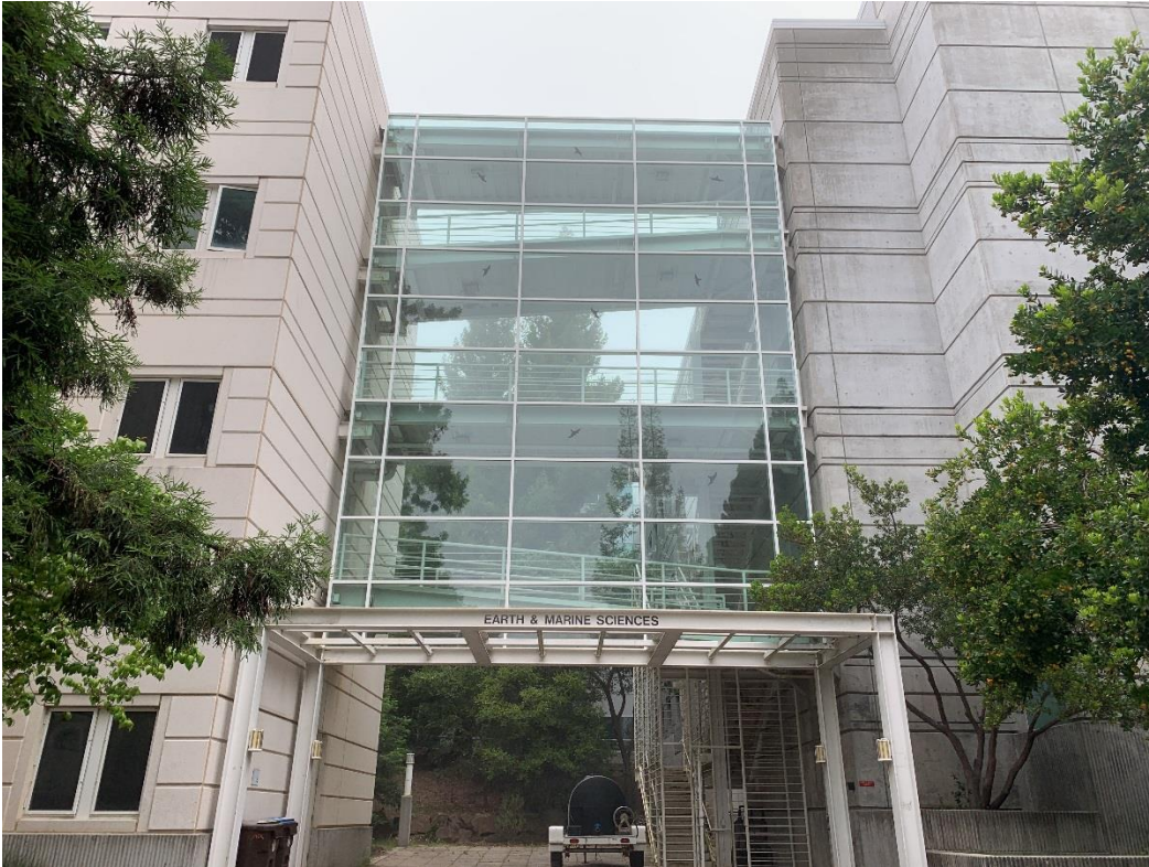
South Elevation Office Block A1 (Left), Bridges ( Center), Lab Block D (Right)
