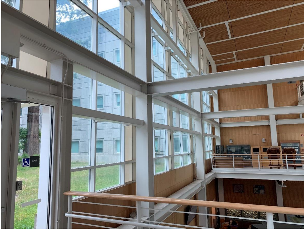
Atrium Interior View at Second Floor (Looking Southwest out to Courtyard)
