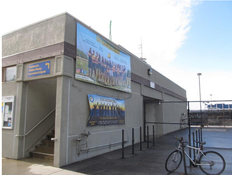
Northwest corner (looking southeast)
