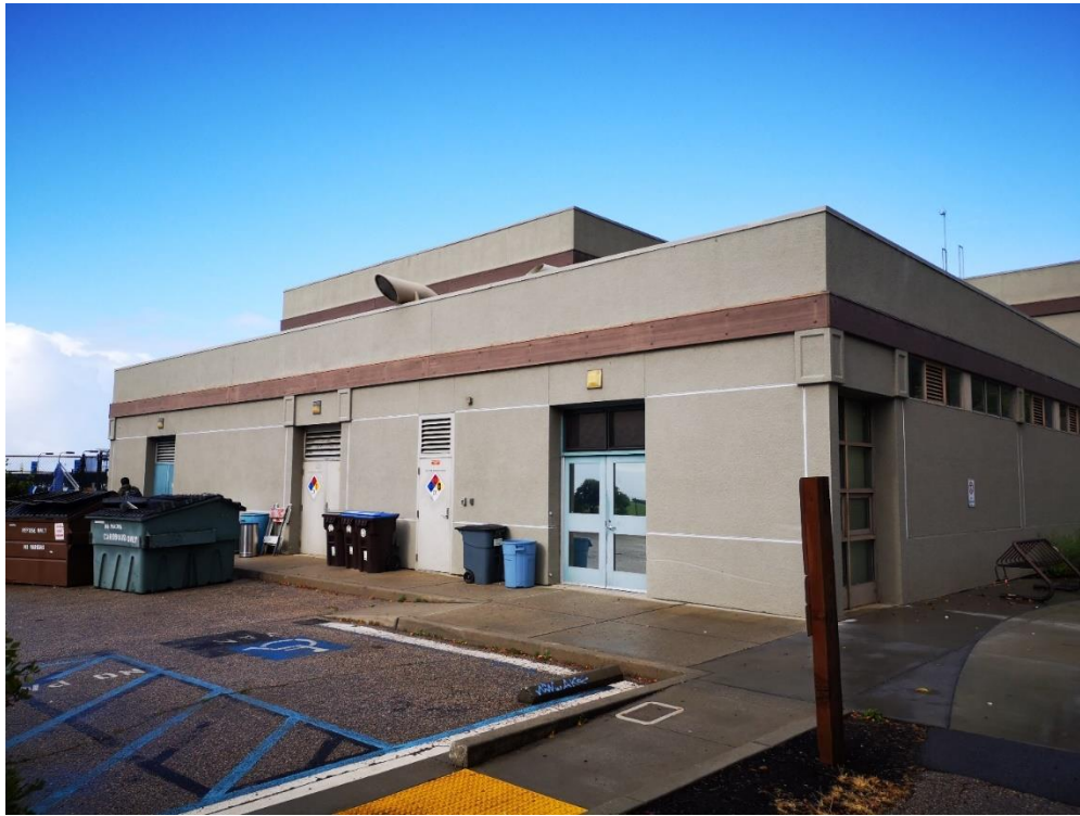
Northeast corner (looking southwest)
