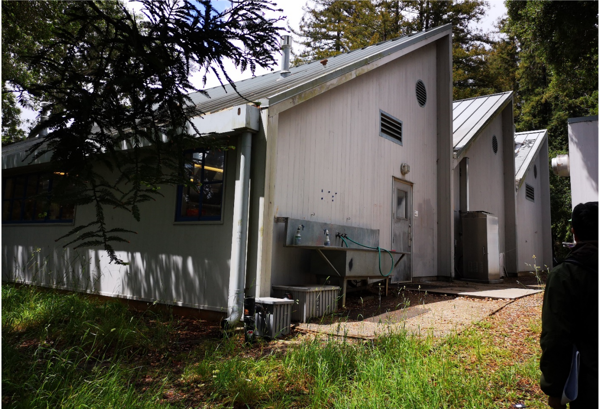
Southeast Corner of Building G (Looking Northwest)
