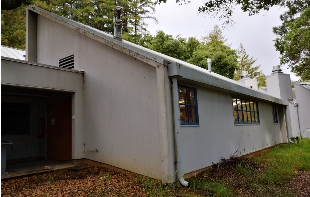
Southwest Corner of Building G (Looking Northeast)
