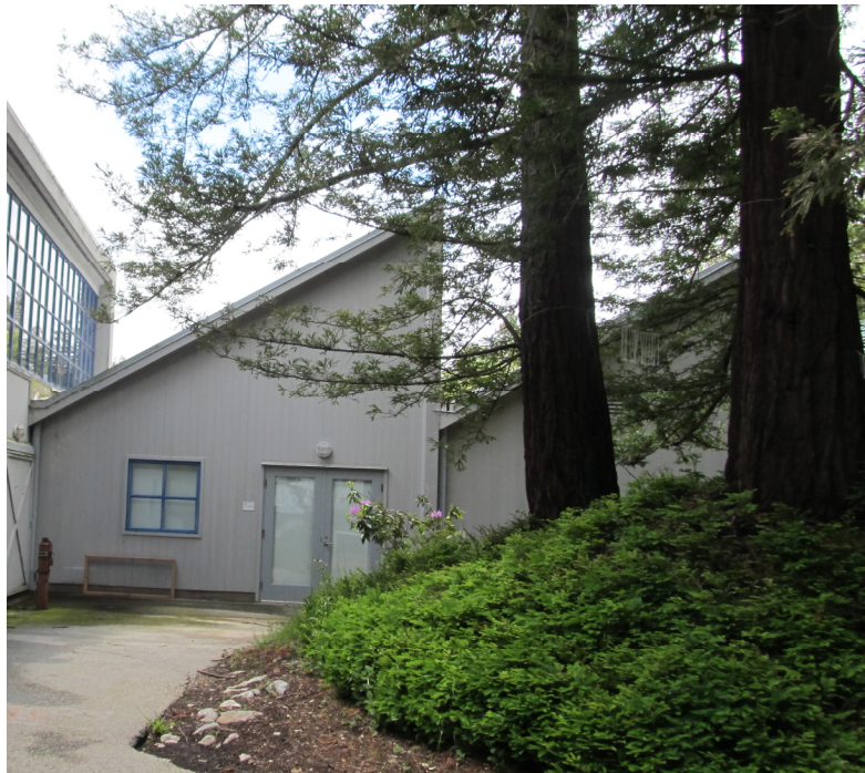
Partial East Elevation of Building F (Looking West)
