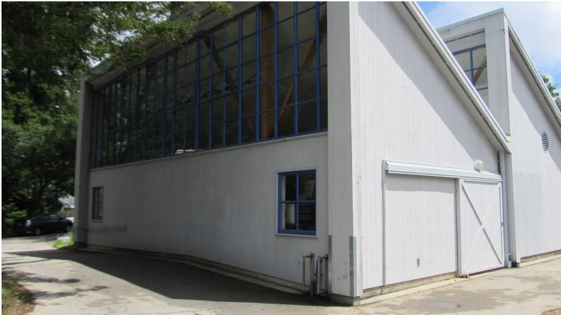
Northwest Corner of Building F (Looking Southeast)
