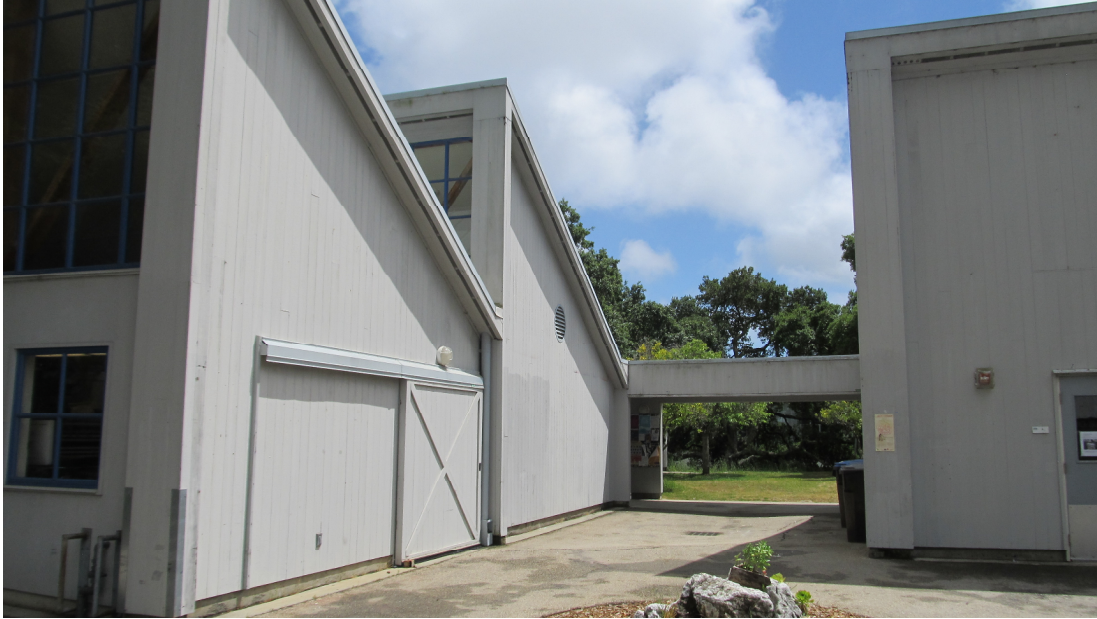
West Elevation of Building F (Looking Southeast)
