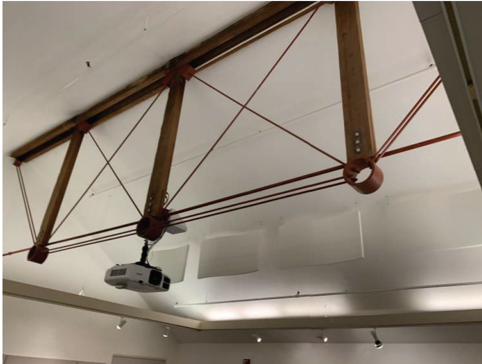
Wood and steel truss below roof
