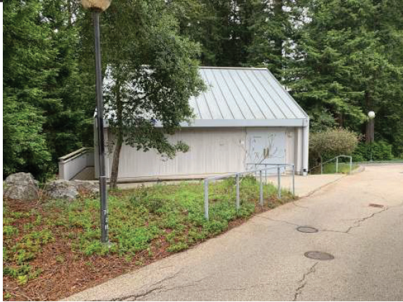
Southwest facade (looking northeast)
