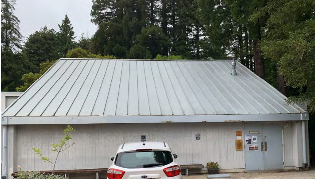
South Elevation (Looking North)
