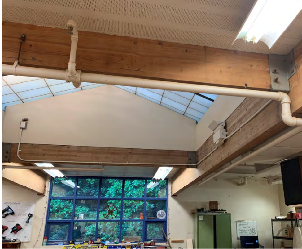
Glulam Beams in the 1996 Addition (Looking North)
