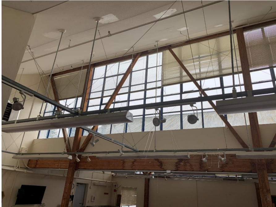
Elevation of Clerestory Window and Braces at Line B (Looking Southeast)
