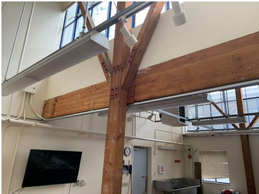
Interior Wood Braced Frame Connection to Glulam Beam at Line B
