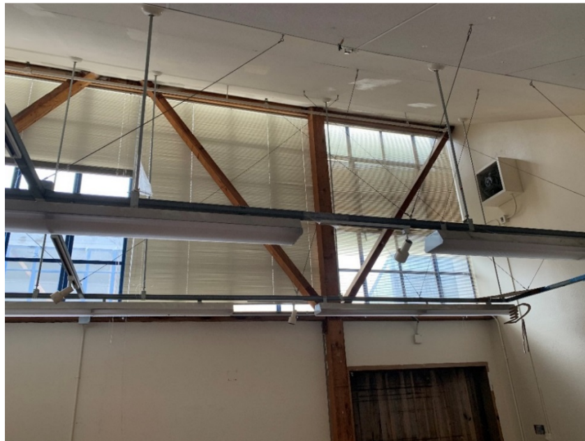
Elevation of Clerestory Window and Braces at Line C (Looking Southwest)
