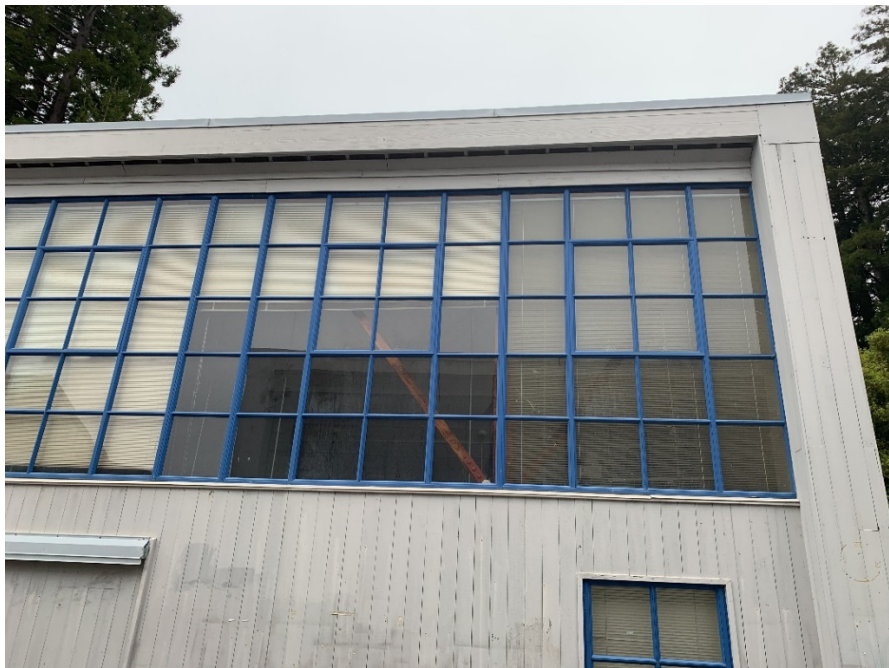
South Elevation of Clerestory Window (Looking North)
