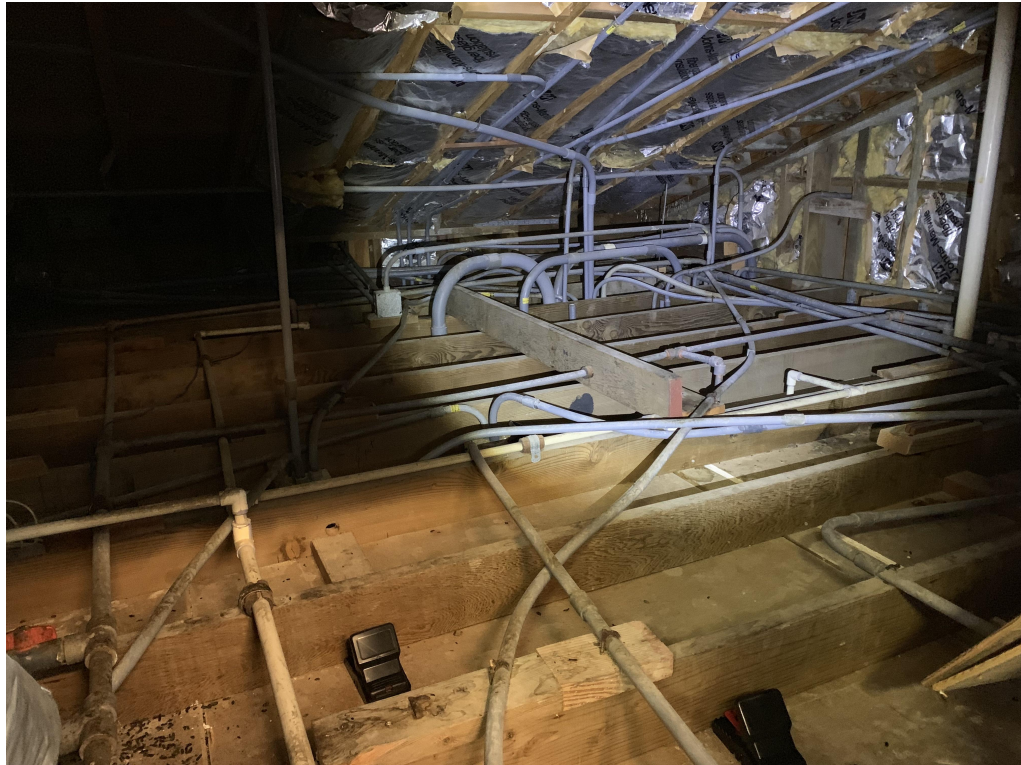
Roof diaphragm framing
