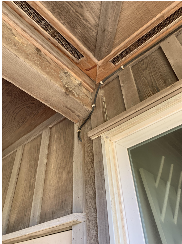
Addition roof connection to original structure
