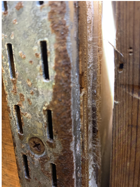
Plywood shear wall behind redwood wall cover
