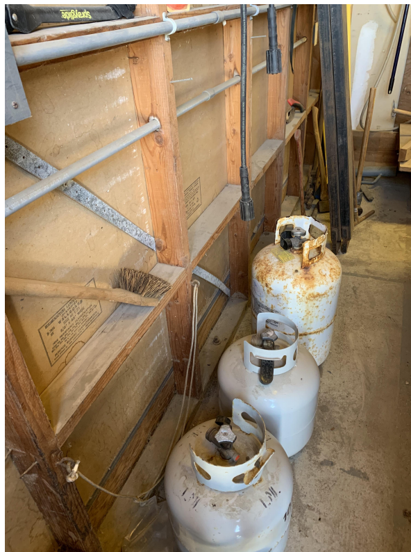
Storage shed metal straps
