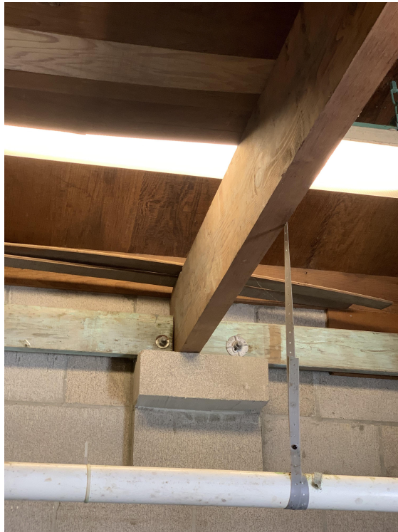
Exterior View and Removable Joist
