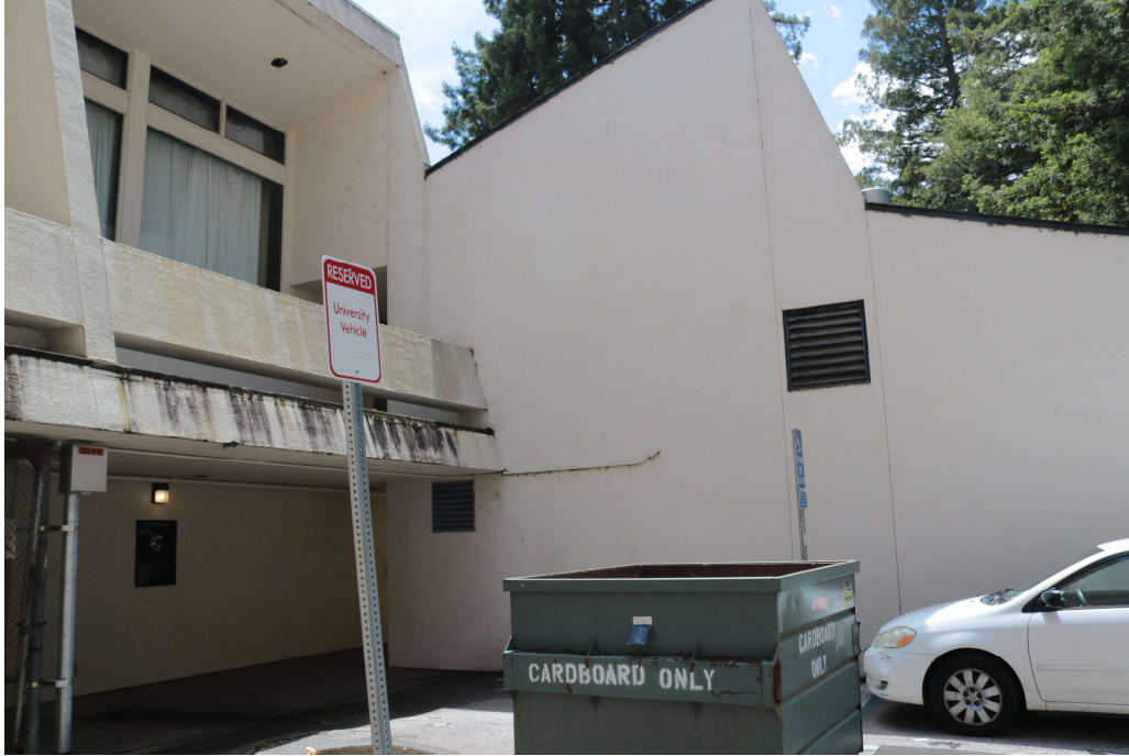
North elevation, showing walkway connection between Building D (CAAN 7314) and Building E (CAAN 7315)
