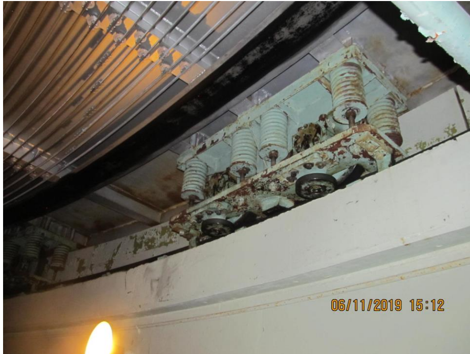
Roller trucks supporting the dome
