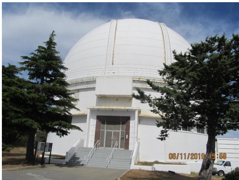
West elevation (main entrance)
