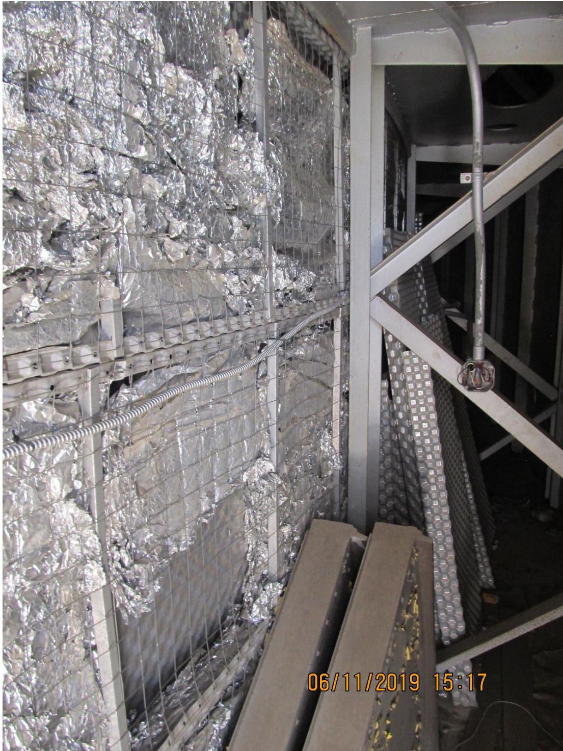
Nonstructural inner wall of the dome
