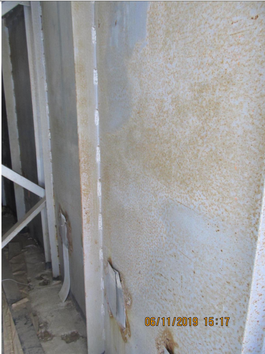
Inside view of the dome with stiffening ribs and periodic trussed ribs
