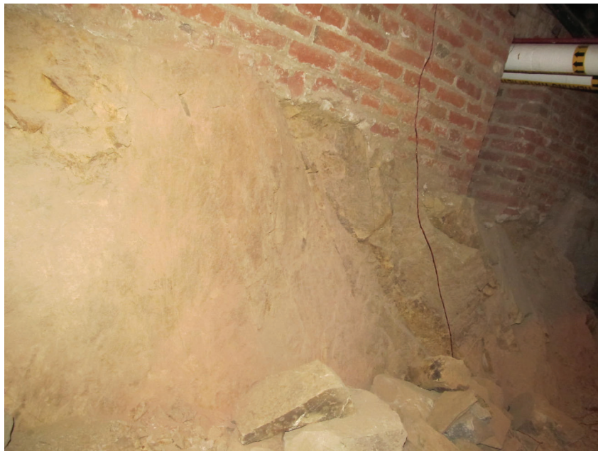
Rock Substrate Directly Under Brick Footings
