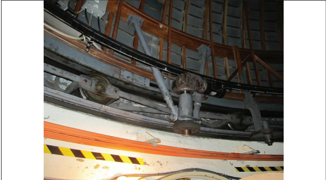
Roller Trucks Supporting the North Dome
