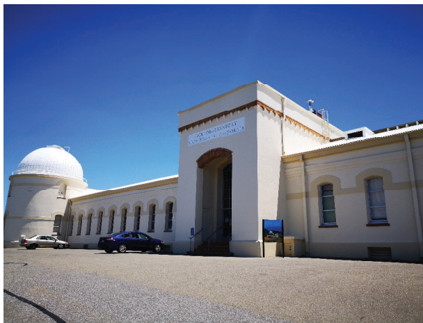
West Elevation (Looking Northeast)
