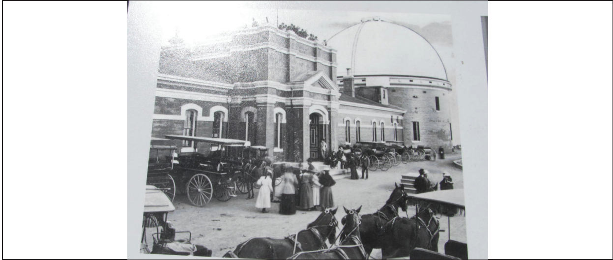
Vintage Photo of the Building (Well) Before Retrofitting Showing Exposed Brick
