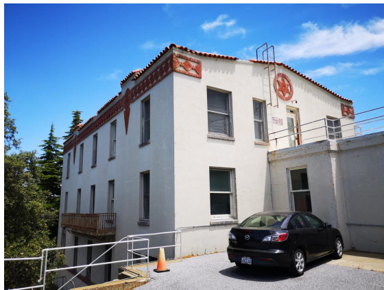
East Elevation (Looking Southeast)
