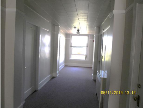
Interior Corridor of Level 3
