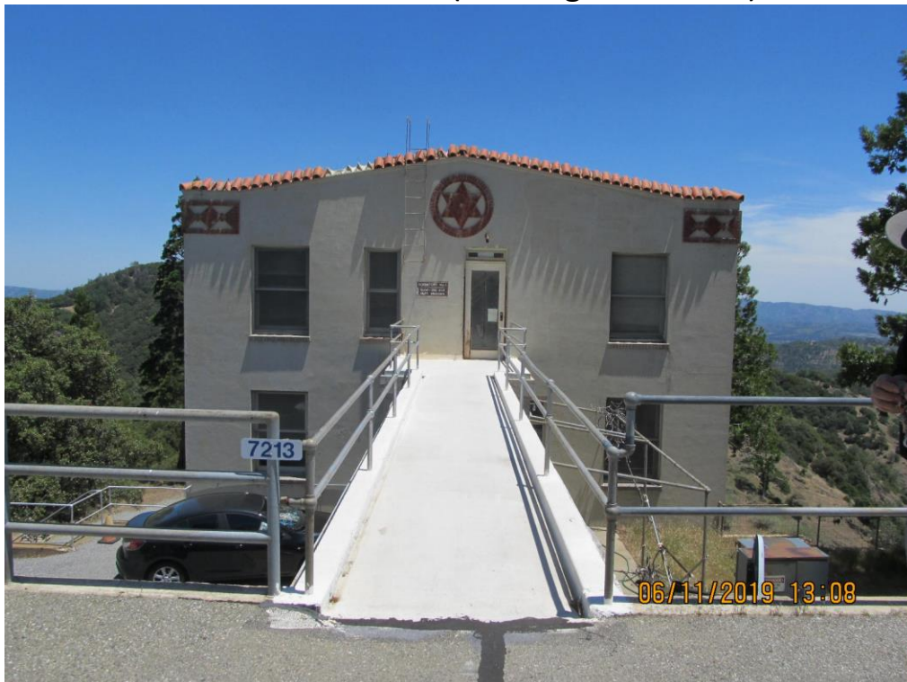
West Elevation (Looking East)
