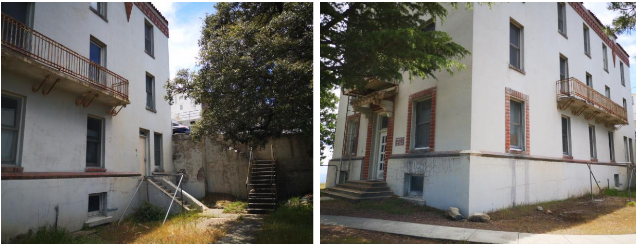
North Elevation (Looking Northwest)
