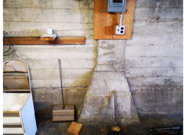
Tapered Column End in Basement
