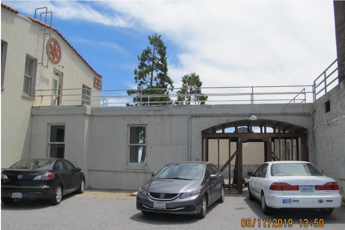
Exit Structure North Elevation (Looking South)
