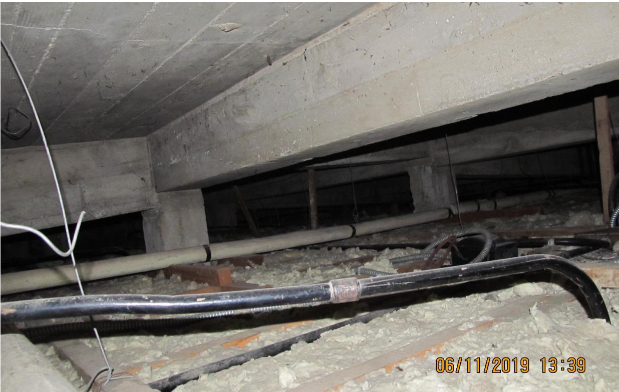
Underside of Roof Structure Above Third Story Ceiling
