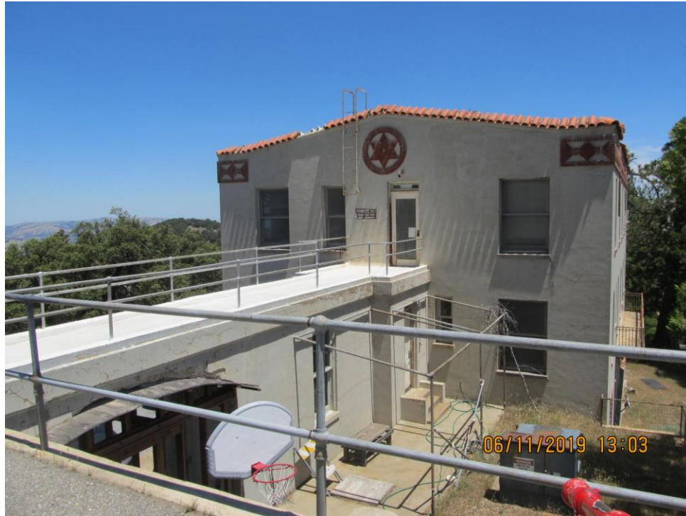
Southwest Corner (Looking Northeast)
