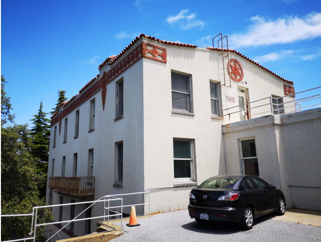
Northwest Corner (Looking Southeast)
