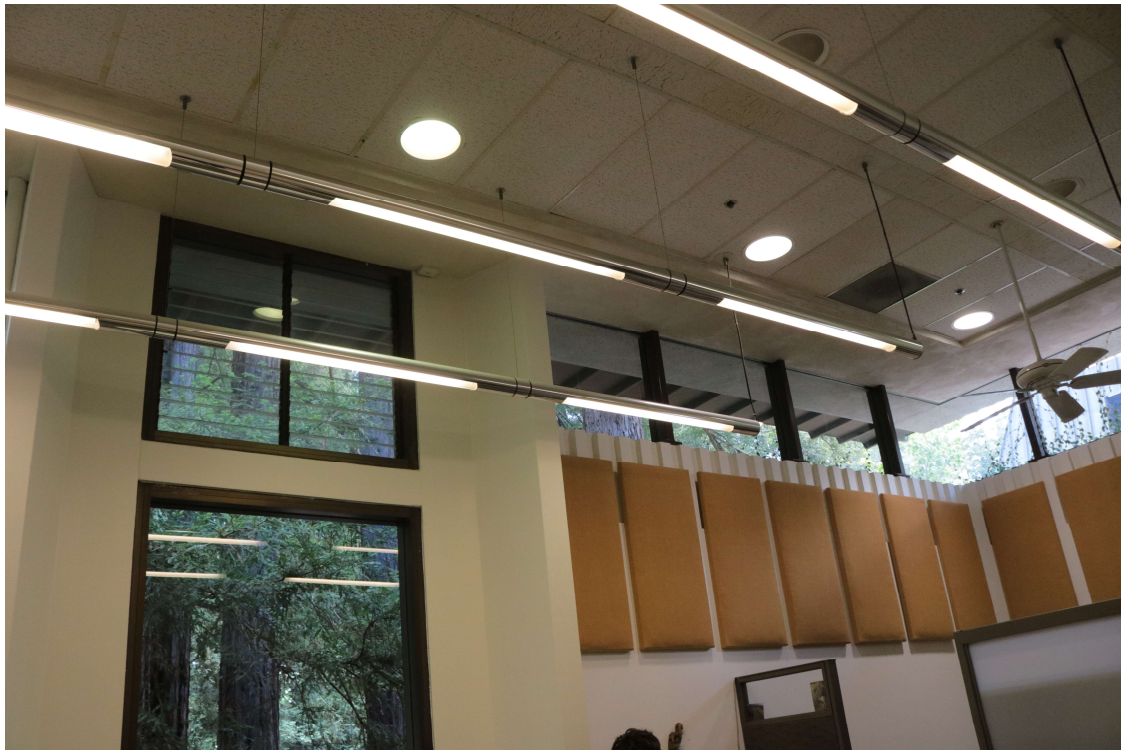
Building interior – precast piers and clerestory windows
