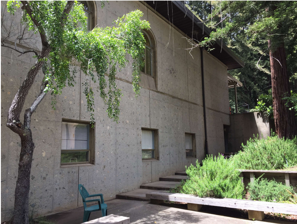
East side of building
