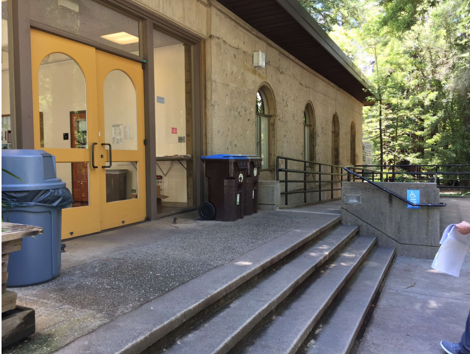
Entry at west side of building
