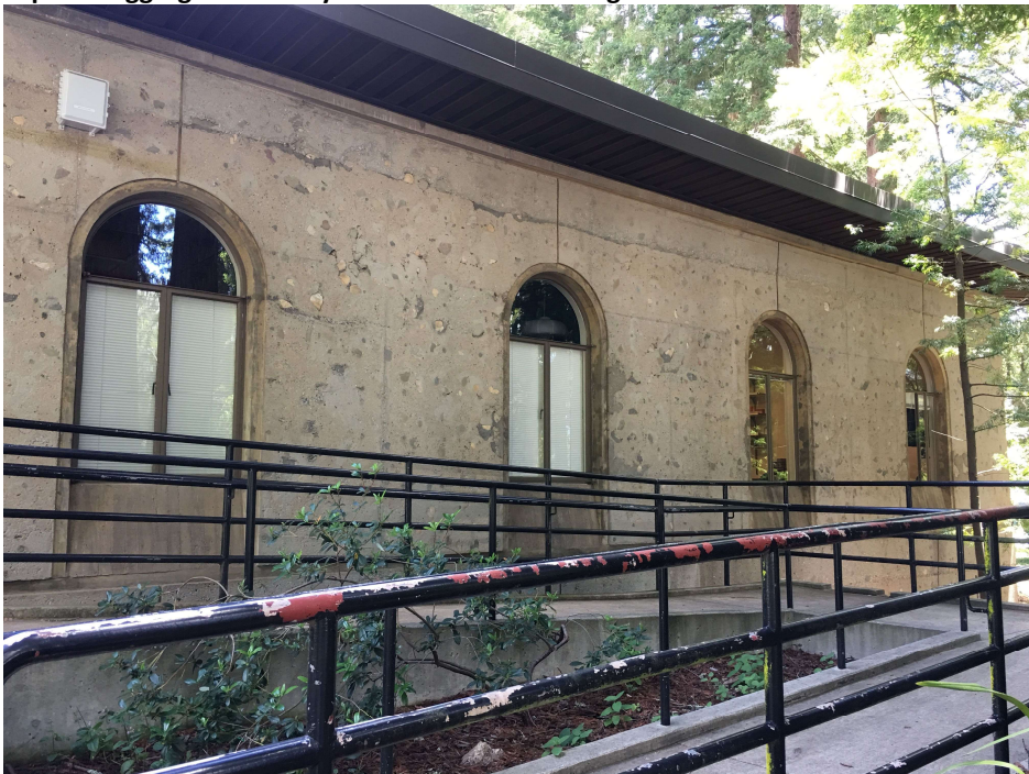
Exposed aggregate at entry at west side of building
