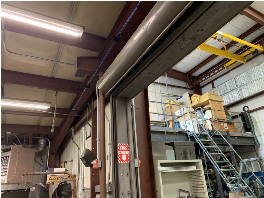
Original structure to eastern addition
