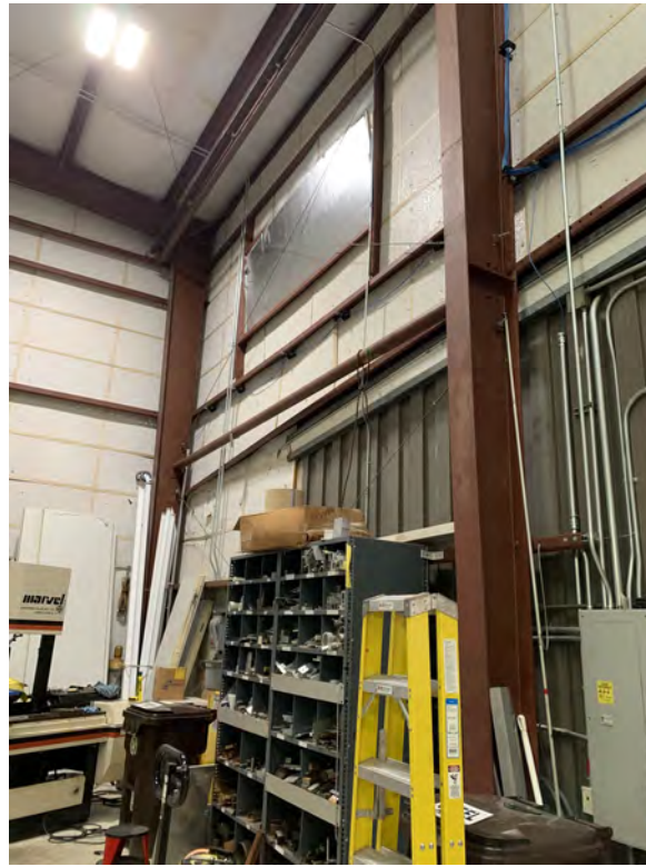
Eastern addition interior
