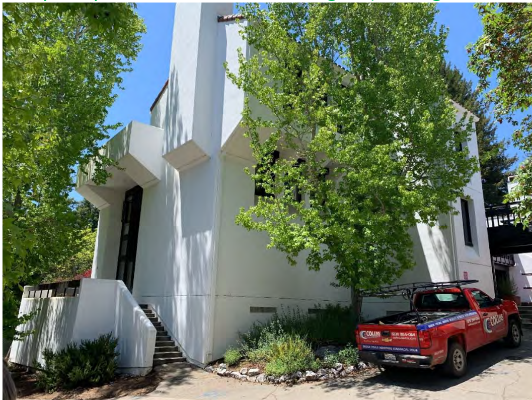
Southeast Corner (Looking Northwest)
