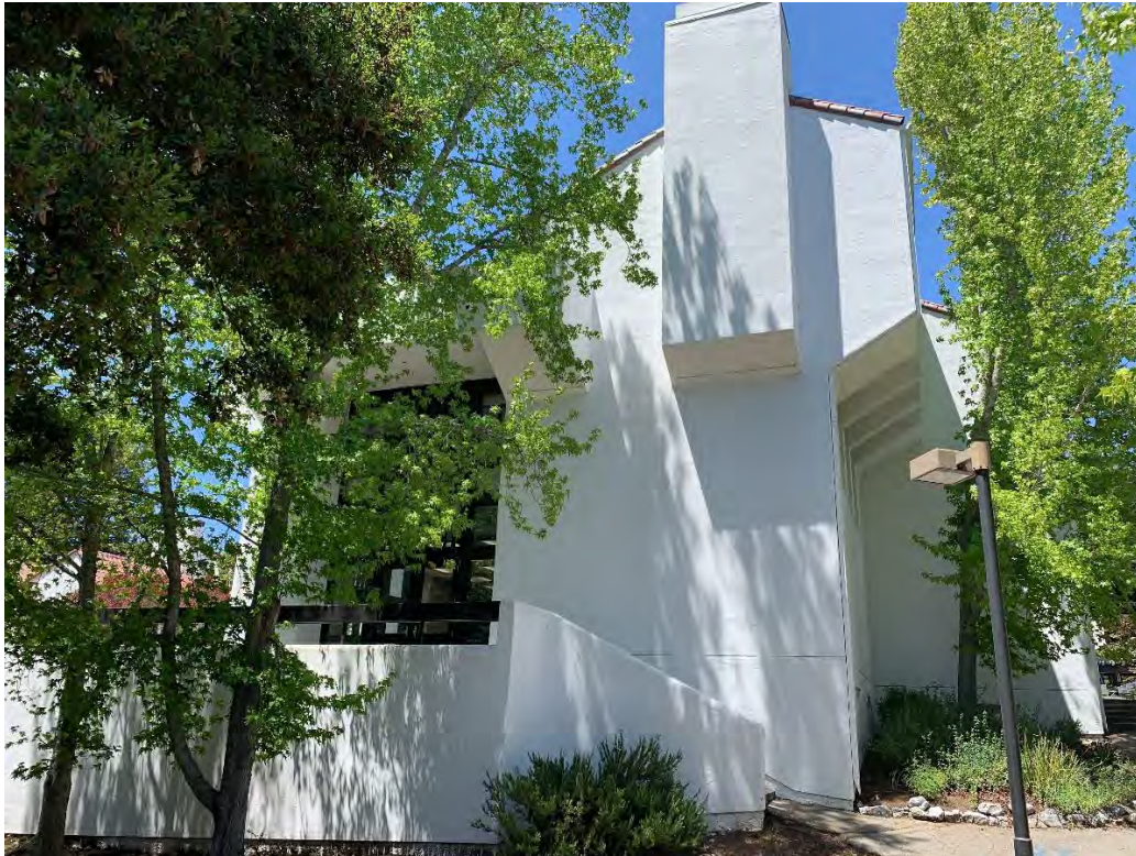
South Elevation with Chimney, Overhanging Floor and Balcony (Looking North)
