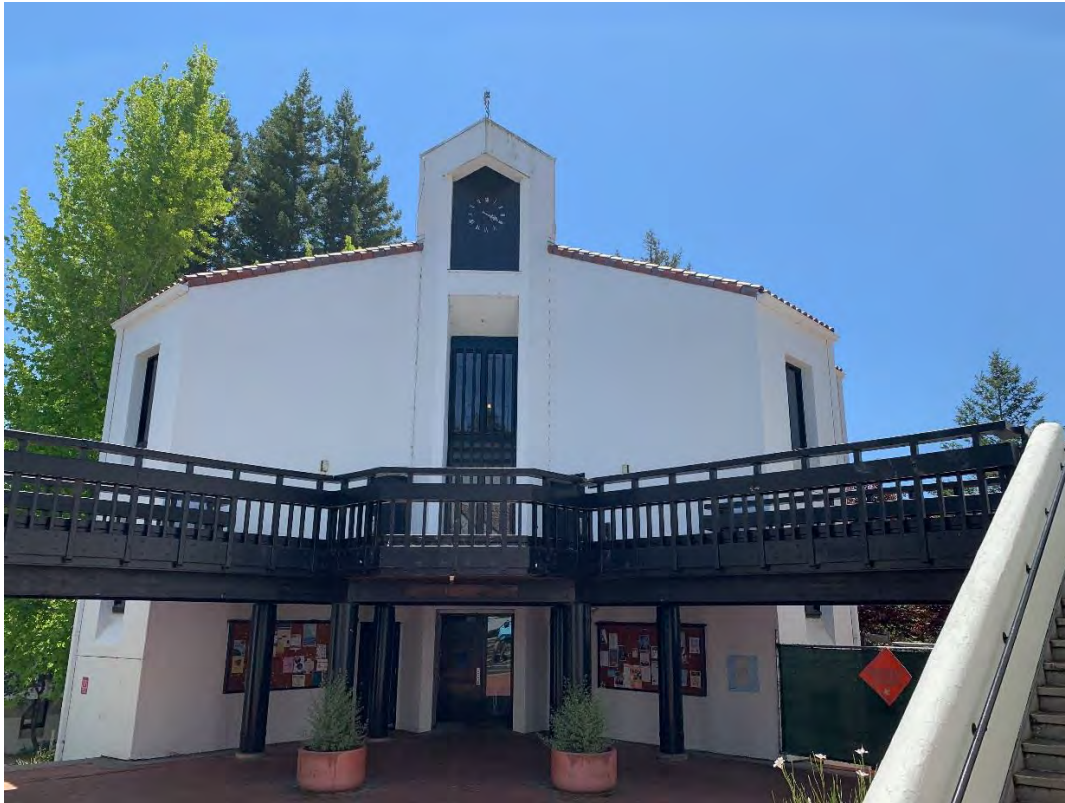
Library Entry with Clock Tower and Pergola (Looking Southwest)
