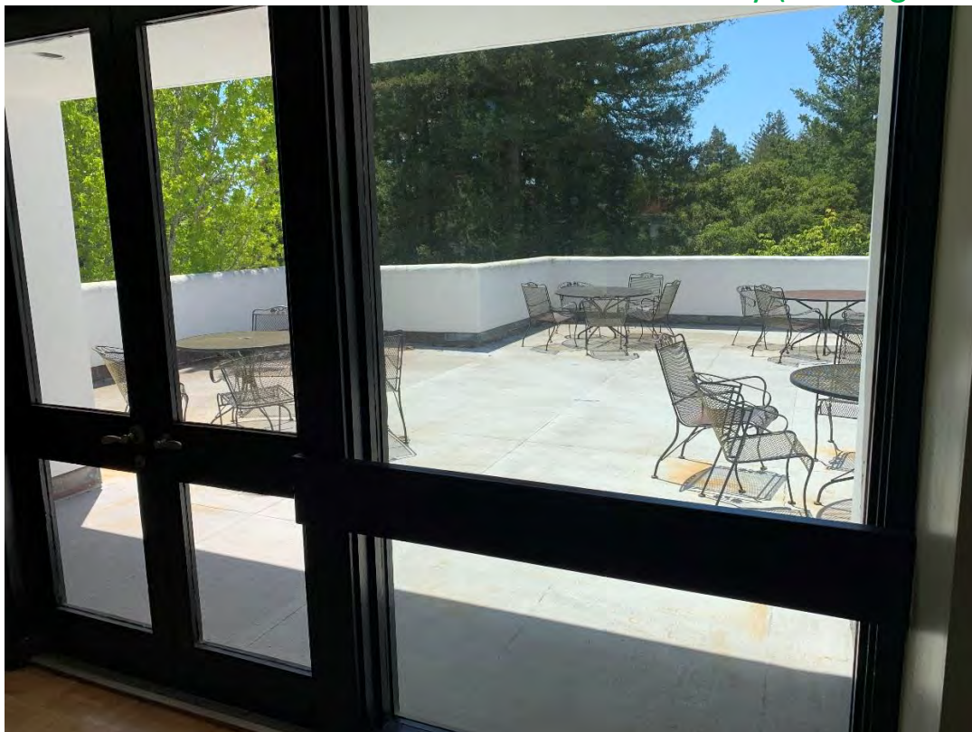
View to Exterior Balcony at Third Floor (Looking Southwest)
