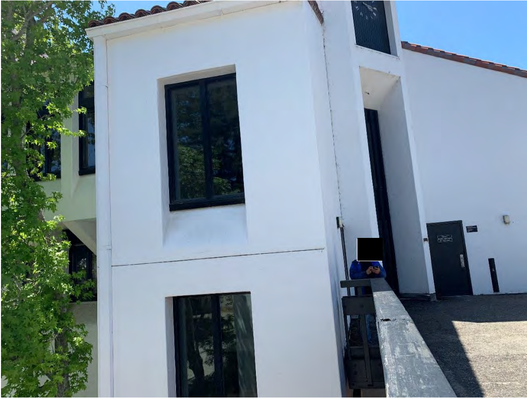
Partial East Elevation from Second Floor Walkway (Looking West)
