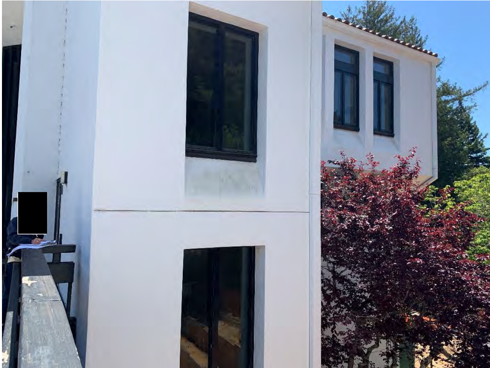
Partial North Elevation from Second Floor Walkway (Looking Southwest)
