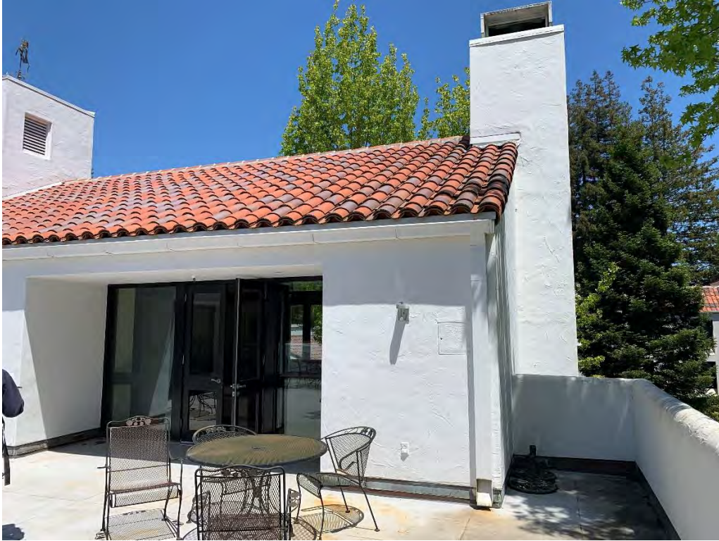
Partial West Elevation at Third Floor from Balcony (Looking East)
