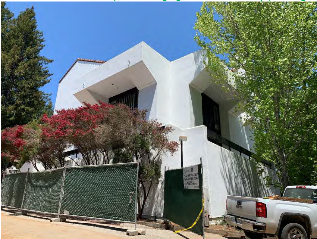
Southwest Corner with Concrete Perimeter Walls at Base and Third Floor Balcony Overhangs on South and West Elevations (Looking Northeast)
