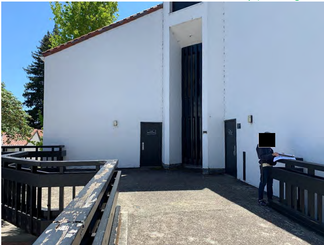
Partial North Elevation from Second Floor Walkway (Looking South)
