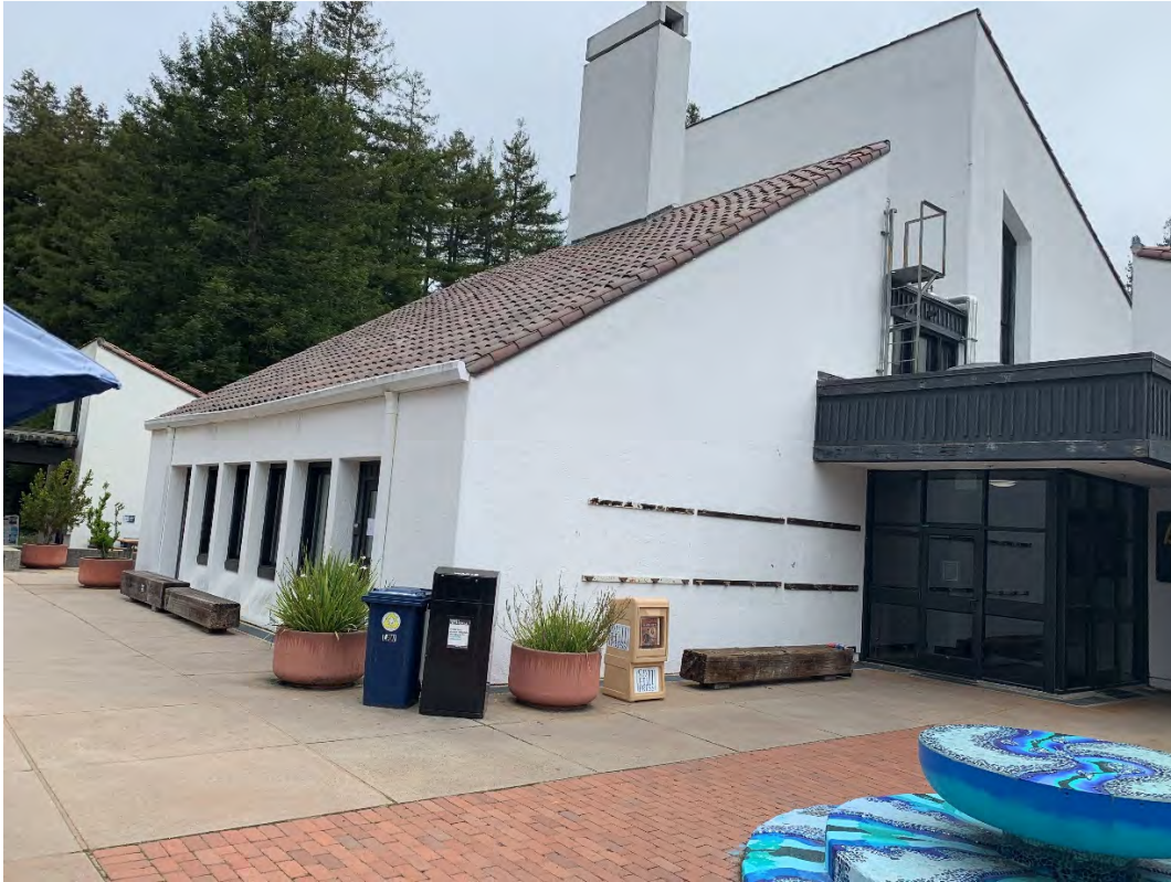
Southwest corner of Fireside Lounge including chimney, glazed entry, and peak of roof above Dining Hall (looking northeast)
