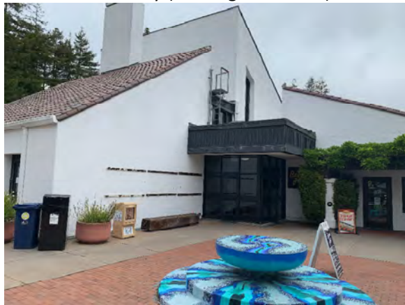
Main Entry (Looking Northeast)
