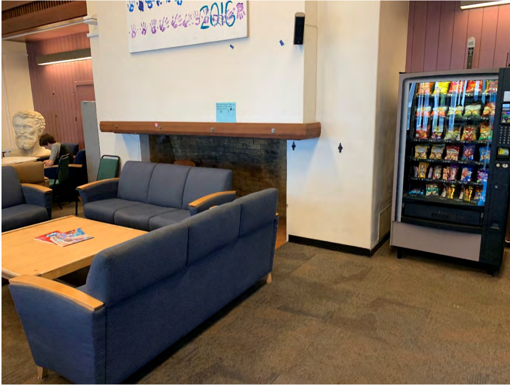
Base of reinforced concrete chimney in Fireside Lounge
