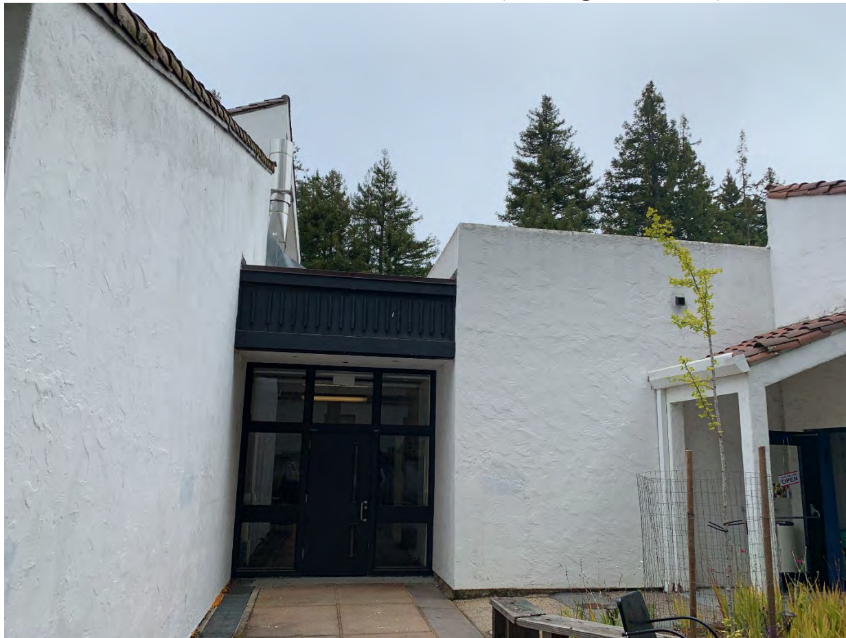
Partial south elevation, Banana Joe's at left, glazed entry and kitchen with flat roof in middle, Merrill College Student Life Wing at right with no visible gap (looking north)
