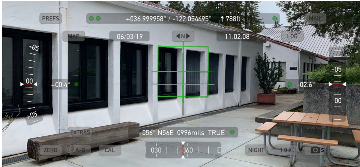
South elevation at Banana Joe's (looking northeast)
