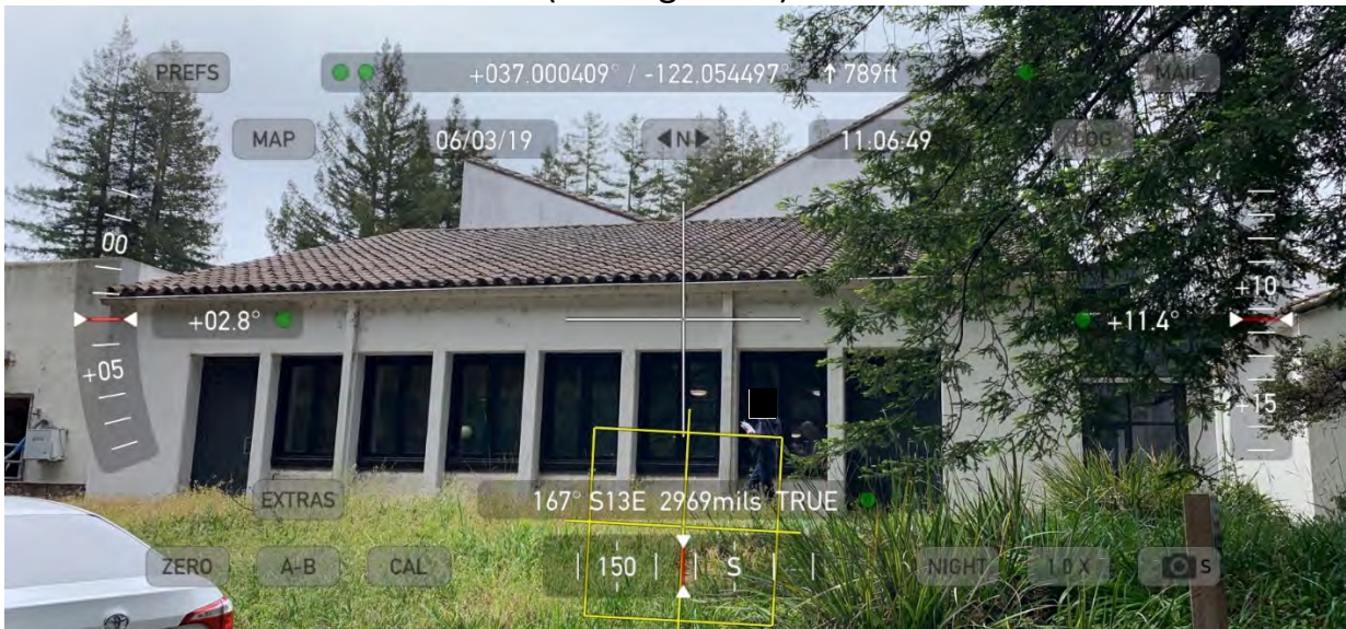
Partial north elevation (looking south)
