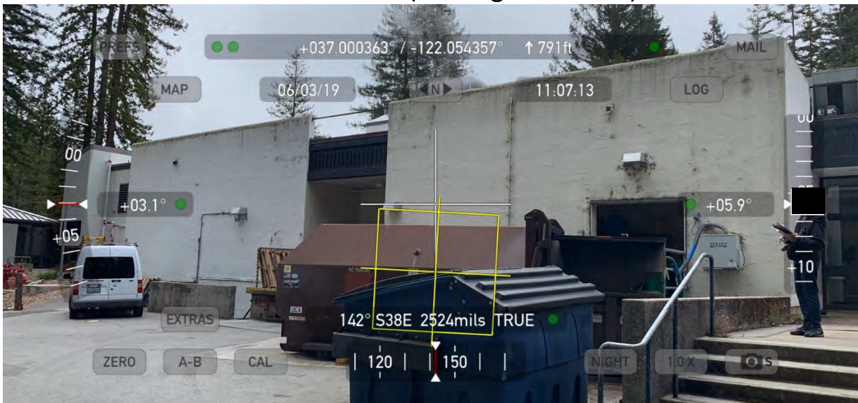
Partial north elevation at Kitchen (looking southeast)
