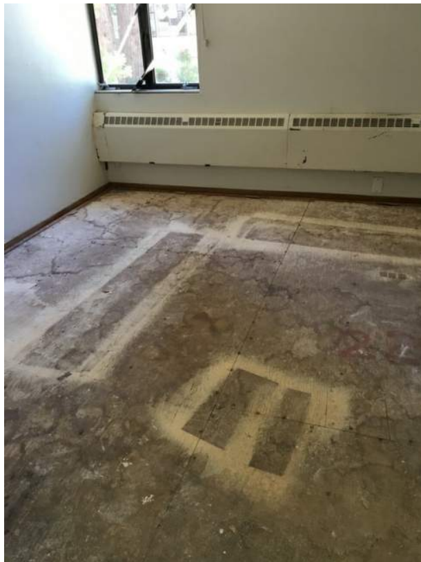
Typical plywood sheathing on building floors
