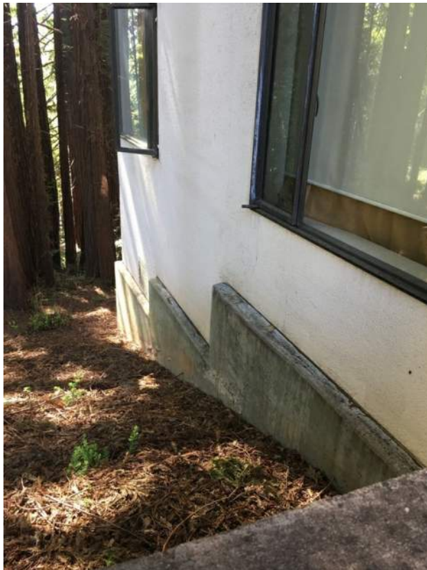
Stepped footing at crawl space
