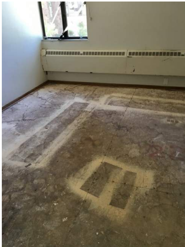
Typical plywood sheathing on building floors
