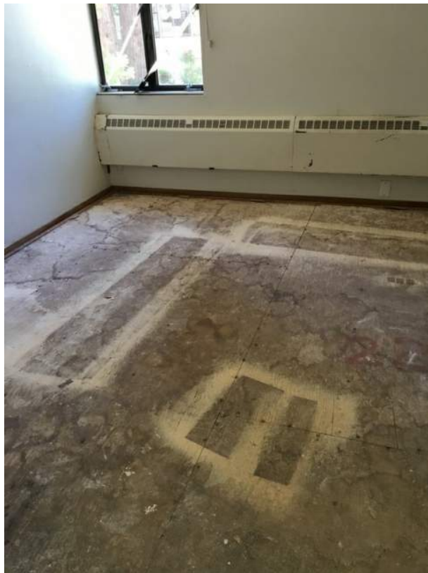
Typical plywood sheathing on building floors
