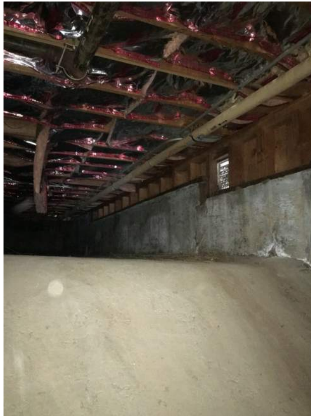
Framing in crawl spaced supported on perimeter retaining walls.
