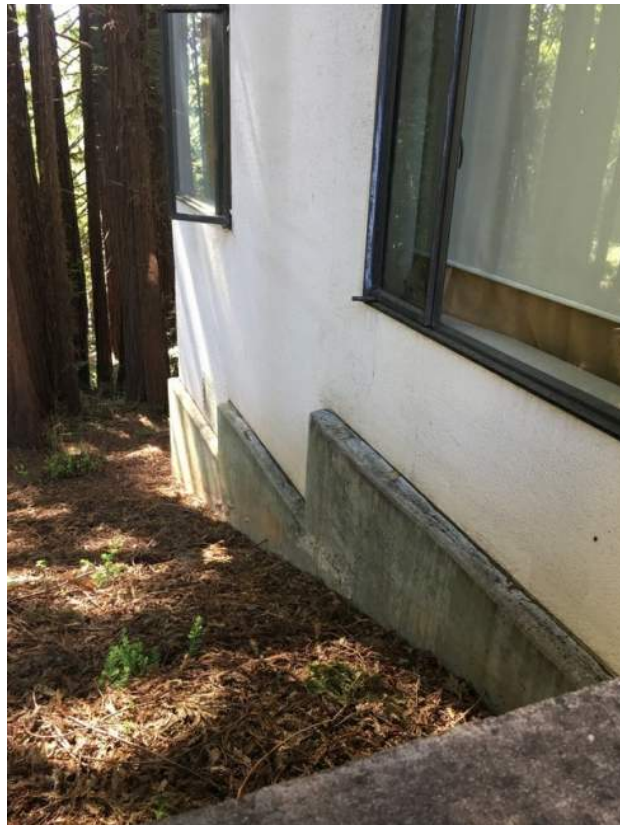
Stepped footing at crawl space
