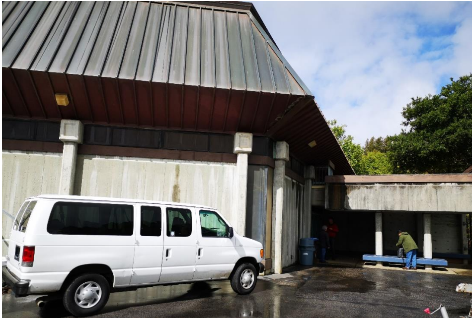
Northeast Corner of General Purpose Room (Looking West From East Lower Grade Level)
