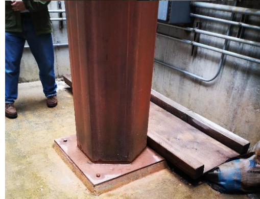
Steel Flues Extending Through Metal Grating and Base Connection
