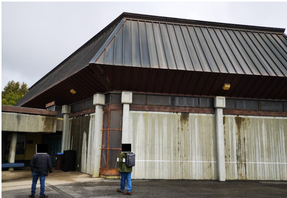
Southeast Corner of General Purpose Room (Looking West from East Lower Grade Level)
