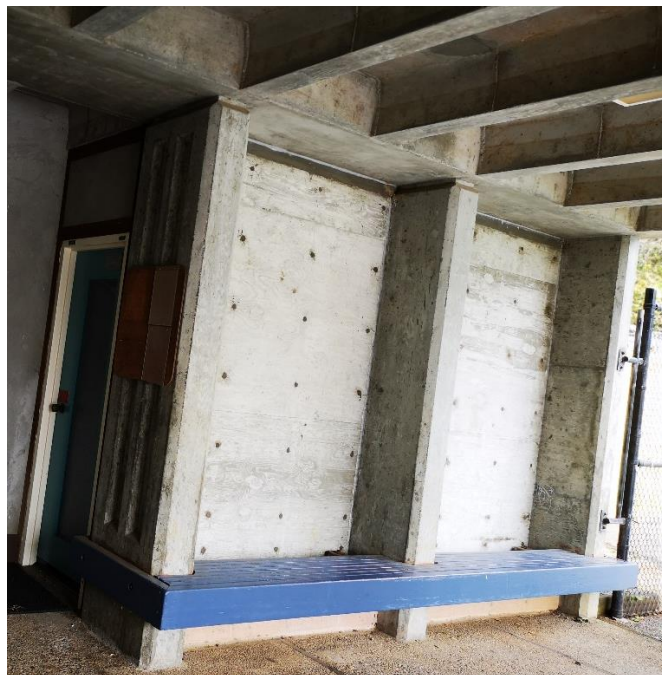
Added Shear Wall in 1988 Seismic Upgrade (Looking Northwest)
