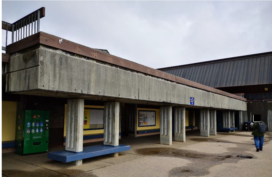
East Elevation of South Rectangular Section (Looking Northwest)
