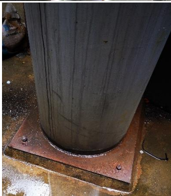
Steel Flues Extending Through Metal Grating and Base Connection
