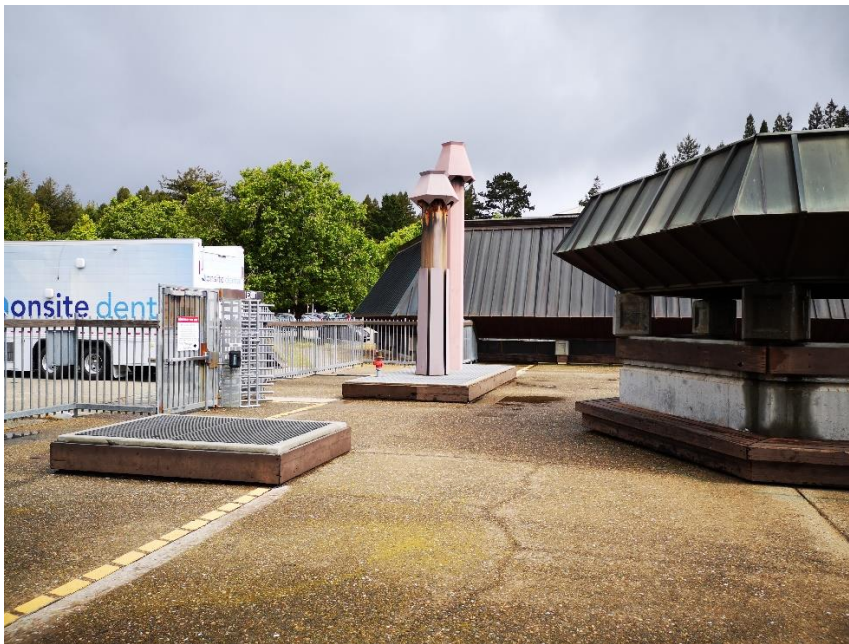
Steel Flues and Stairwell Canopy (Looking North from South Roof Terrace)
