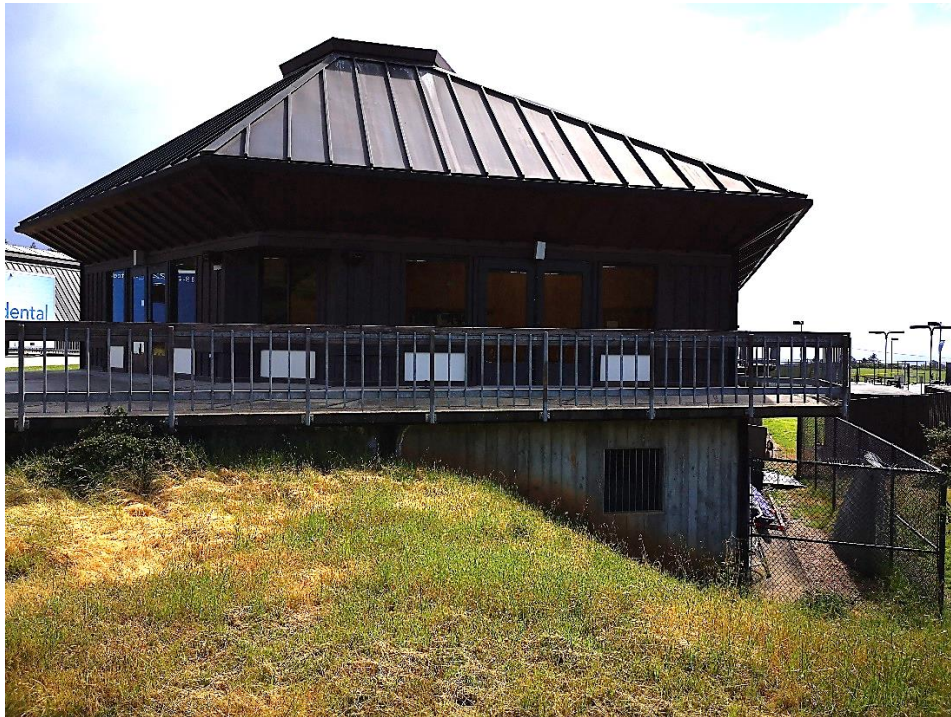
West Elevation (Looking East)
