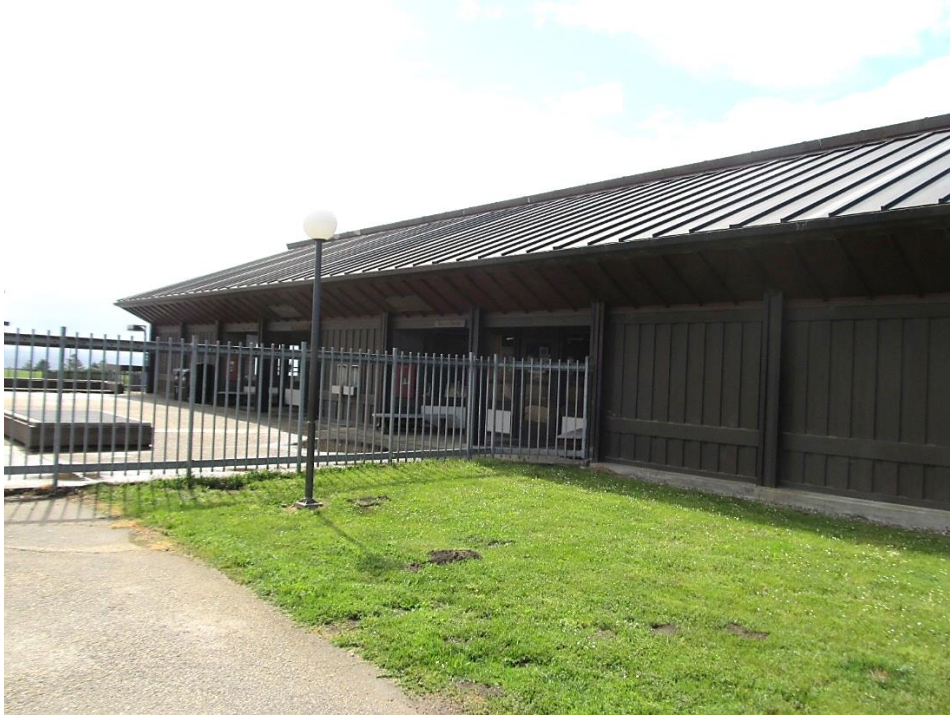
Partial North Elevation (Looking Southeast)
