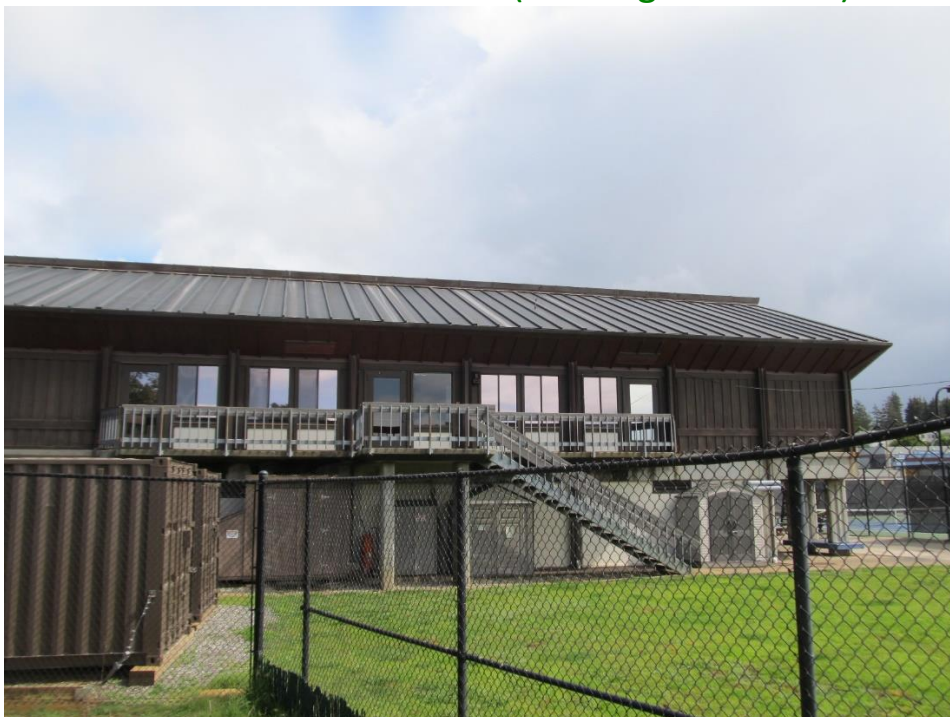
Partial South Elevation (Looking North)
